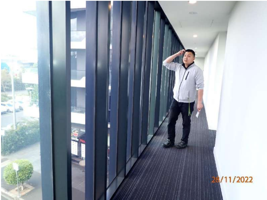
Photograph 81 – Level 4 south passageway aluminium windows
