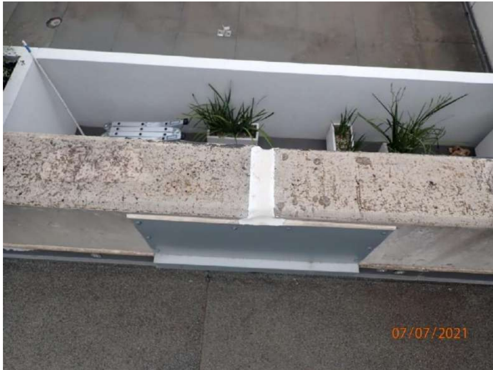
Photograph 121 – Metal plates fixed to large gaps between concrete wall panels on building B roof
