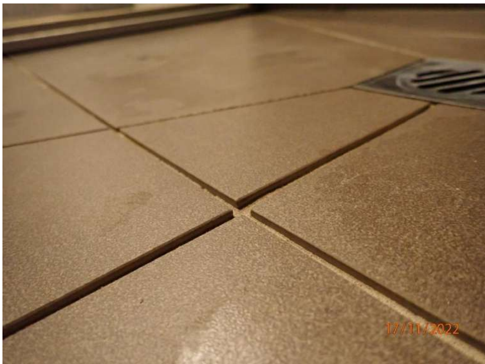
Photograph 8 - Apartment 309A bathroom shower recessed grout lines
