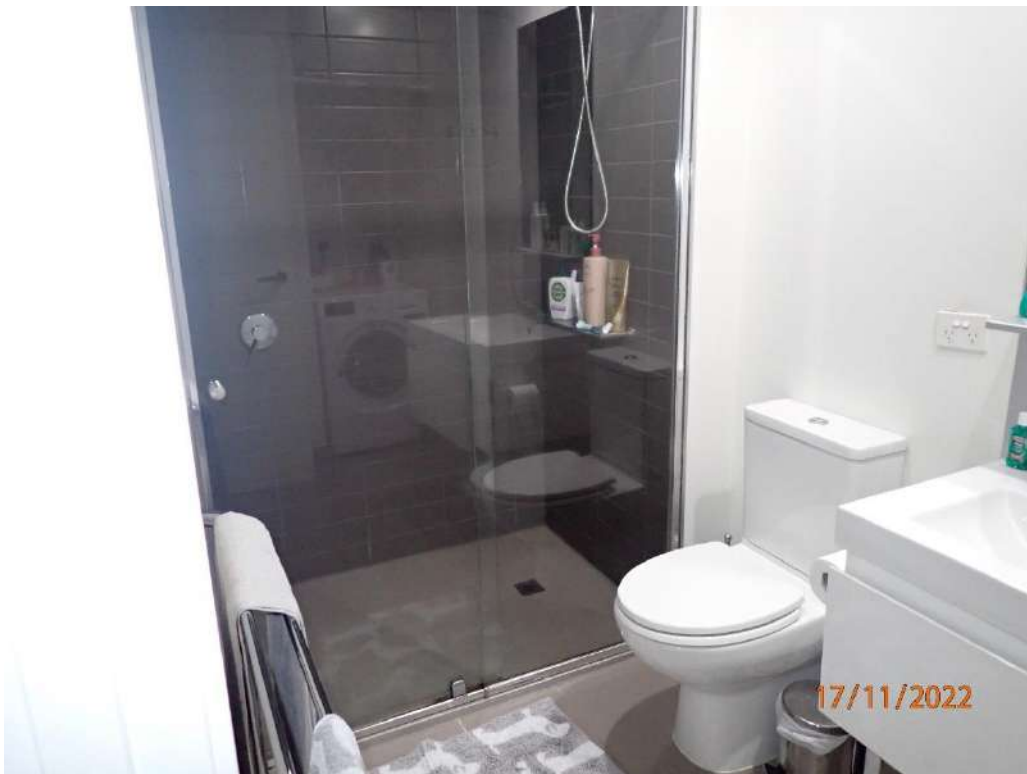
Photograph 32 – Apartment 328B bathroom shower
