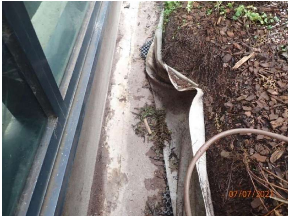
Photograph 83 – Internal waterproof membrane to planter box
