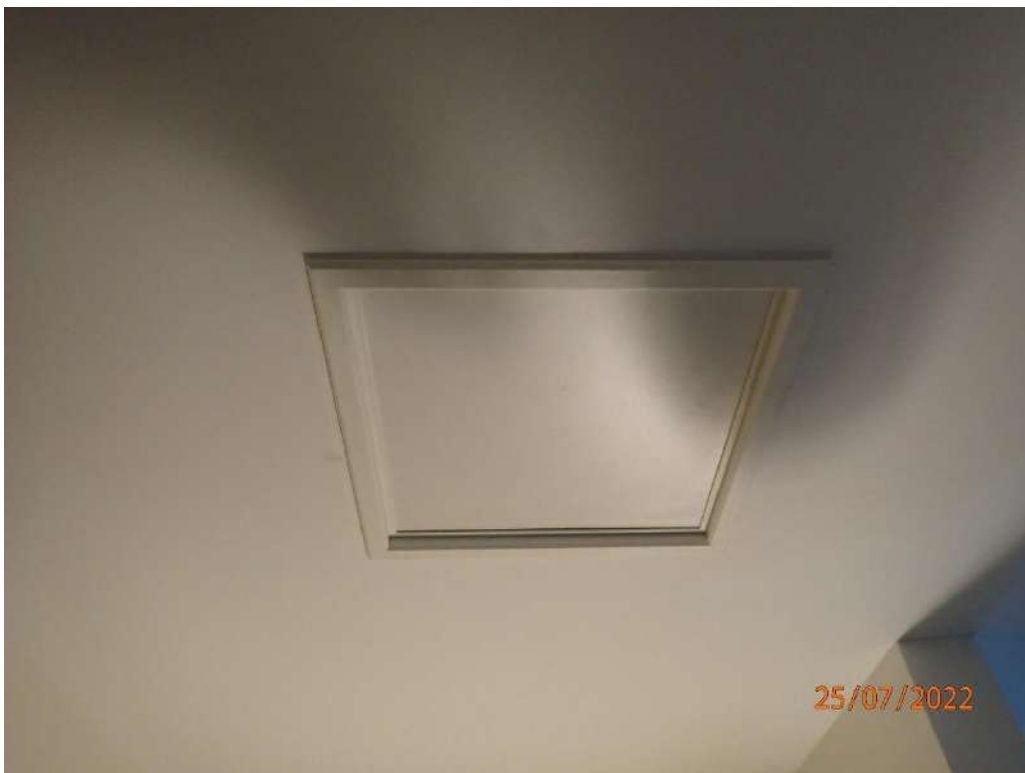
Photograph 168 – Lot 312A/Apartment 312A, entrance hallway ceiling hatch
