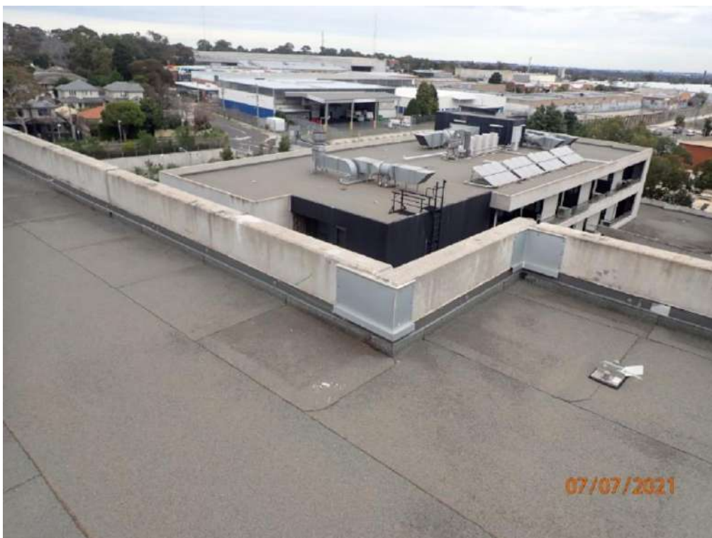
Photograph 120 – Metal plates fixed to large gaps between concrete wall panels on building B roof
