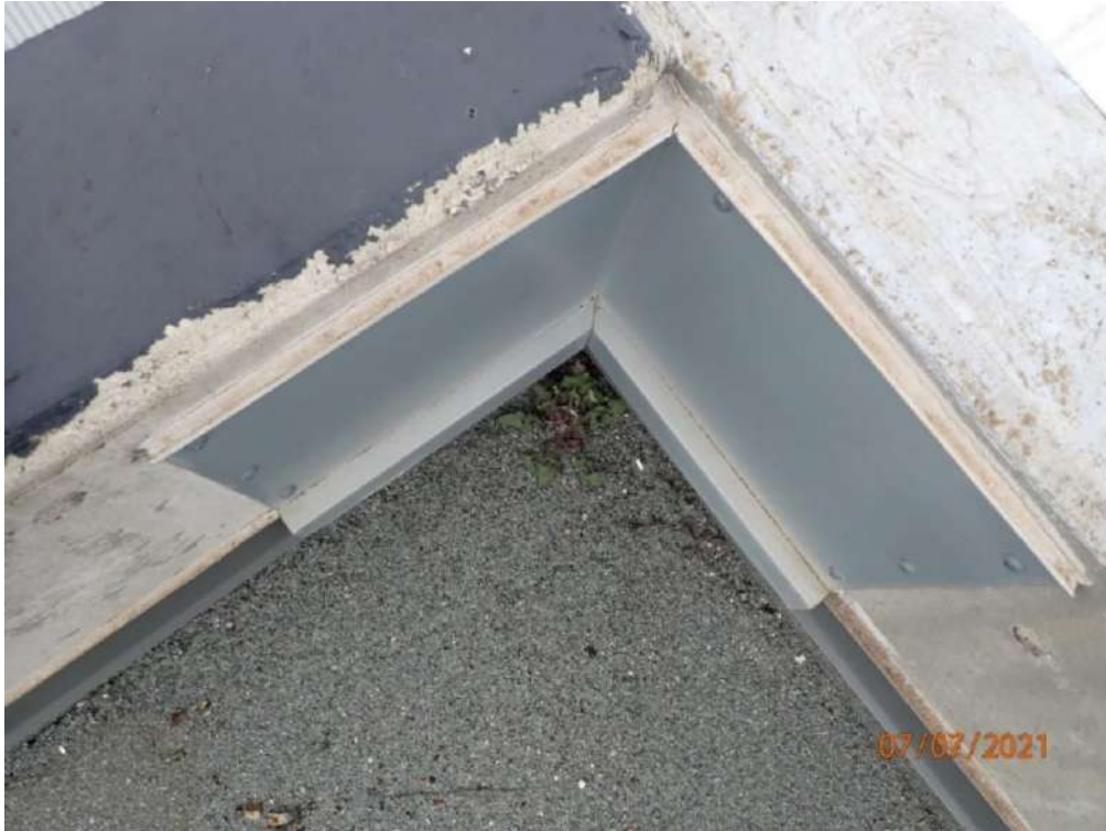
Photograph 123 – Metal plates fixed to large gaps between concrete wall panels on building B roof
