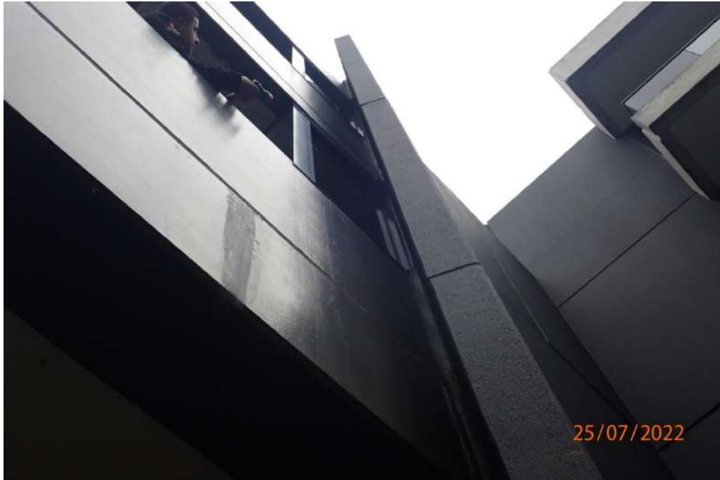
Photograph 182 – Lot 324B/Apartment 336B, water testing to north west apartment windows
