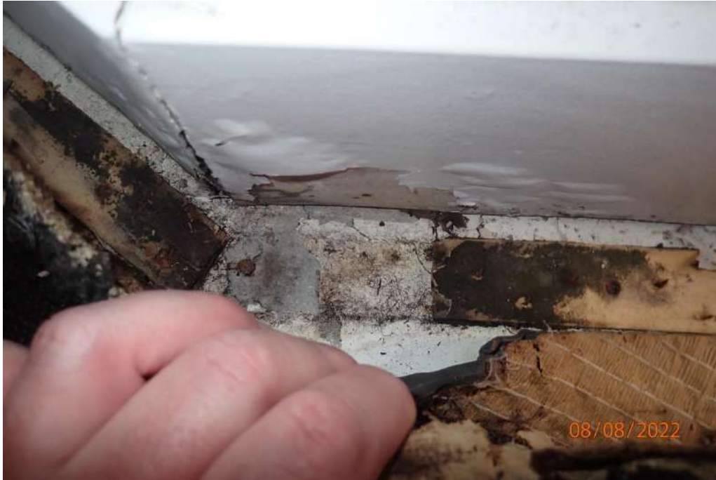
Photograph 187 - Lot 402A/Apartment 402A living area west wall carpet and smooth edge
