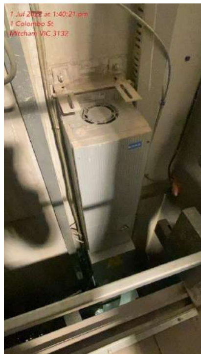
Internal lift shaft, slurry to lift drive
