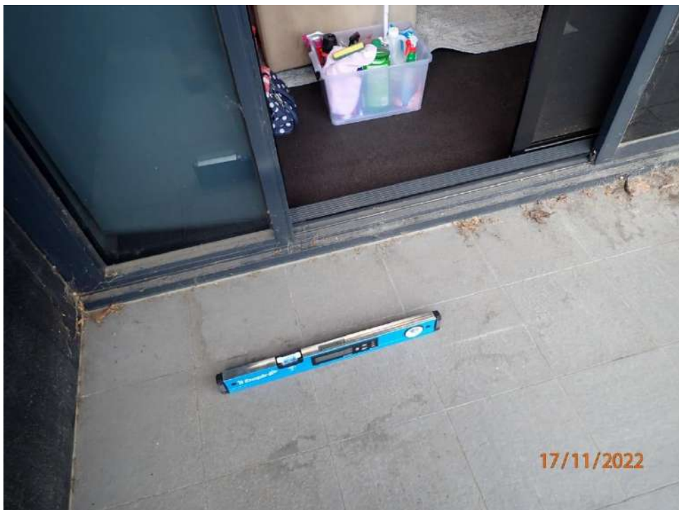
Photograph 10 - Apartment 308A balcony
