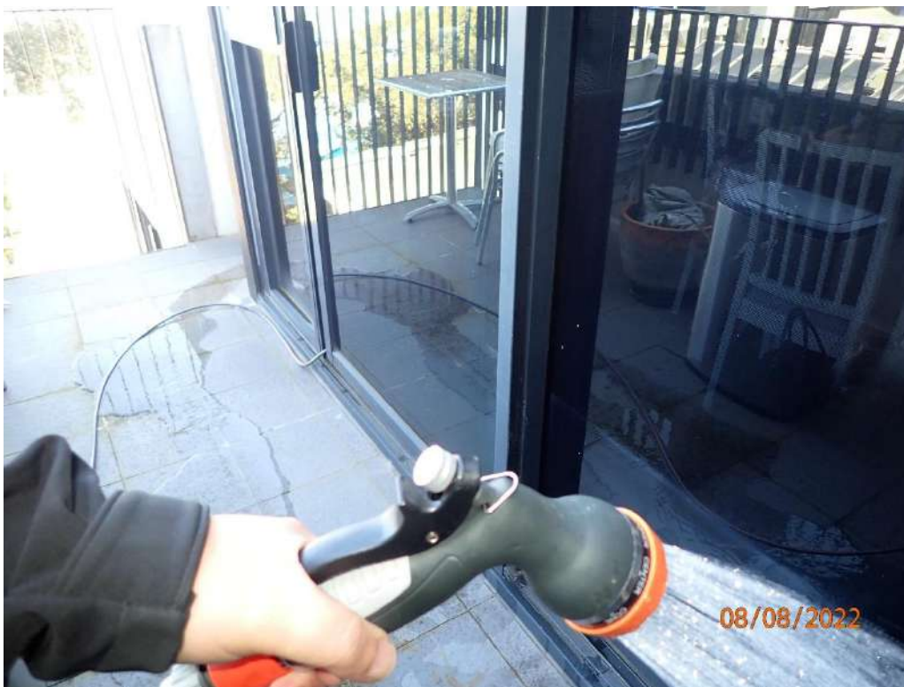
Photograph 214 - 704B/Apartment 703B, water testing to living sliding door opening to balcony
