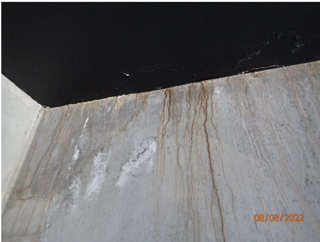
Photograph 134 - Building A north east corner and the centre of the ceiling of the stairwell at the rooftop level
