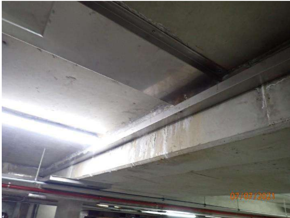
Photograph 53 - Drip tray installed to basement carpark below areas of efflorescence and calcium build up
