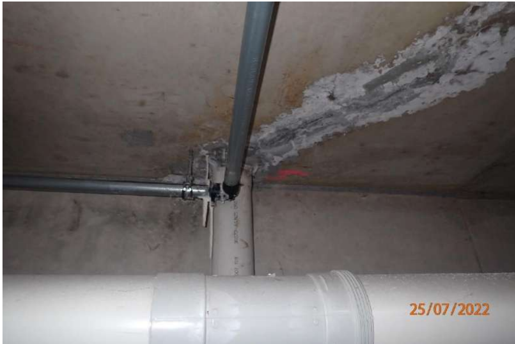
Photograph 153 – Upper basement level, beneath Lot 110A/Apartment 110A planter boxes
