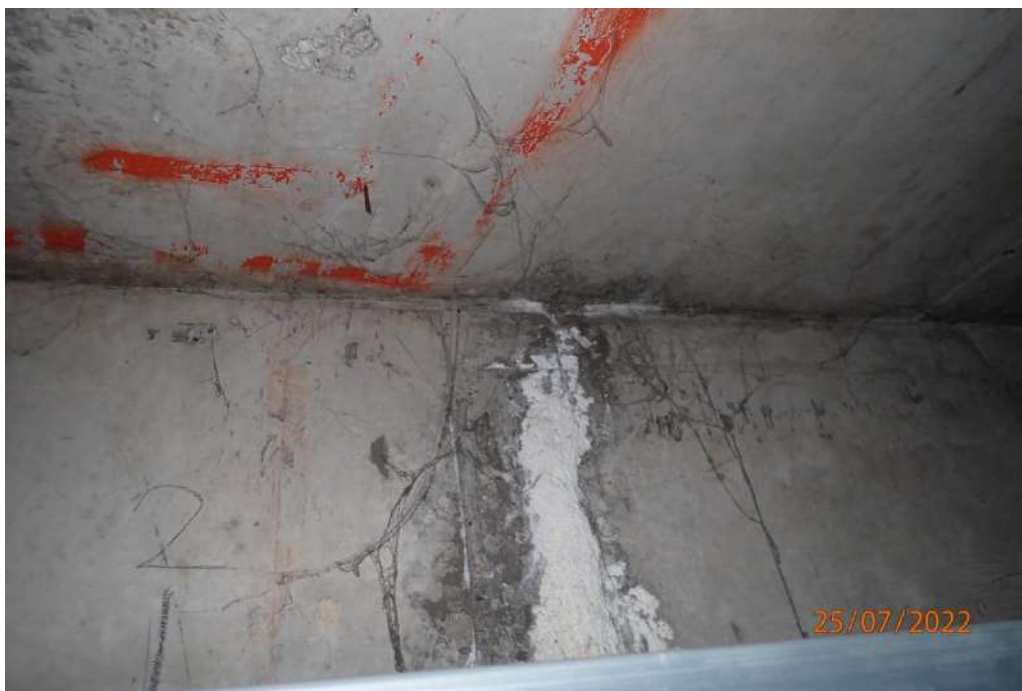
Photograph 150 - No evidence of a drainage point
