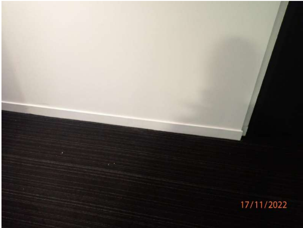
Photograph 41 – Common passageway outside Apartment 328B
