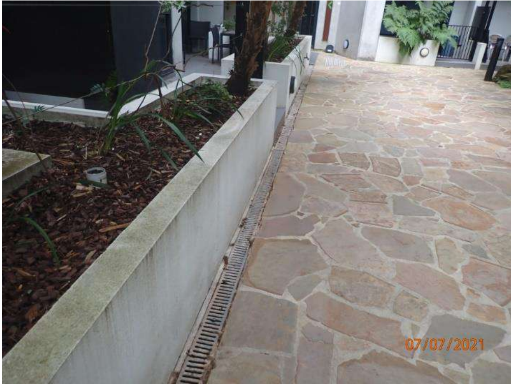
Photograph 69 - Planter boxes to the ground floor courtyards and private lot planter boxes
