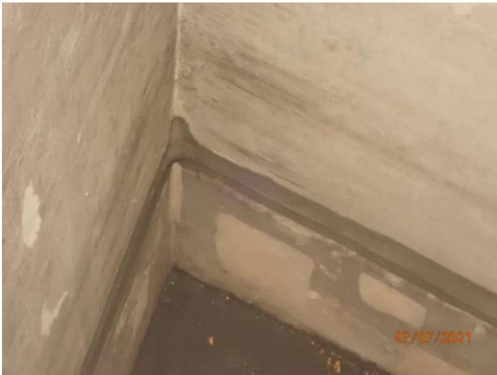
Photograph 90 – Waterproofing and sealant applied to water tank
