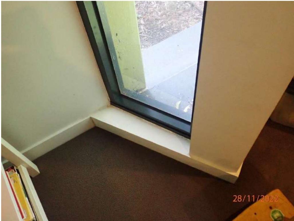
Photograph 67 - Apartment 109A bedroom 2 west window
