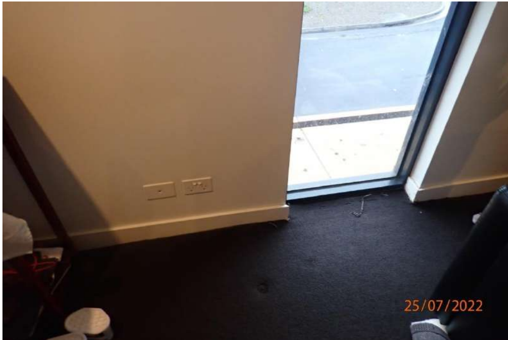
Photograph 173 - Lot 321B/Apartment 333B, single window on the south wall of the living area
