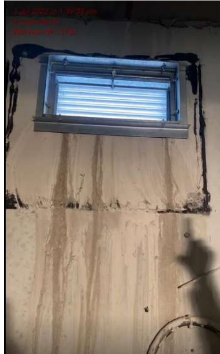
Video snippet 221– internal lift shaft, slurry to internal wall lining
