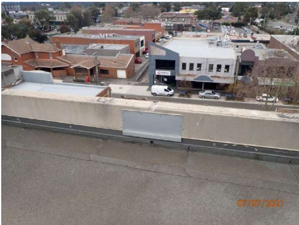
Photograph 124 – Metal plates fixed to large gaps between concrete wall panels on building B roof
