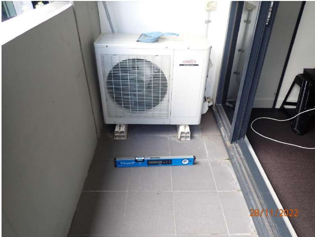
Photograph 95 - Apartment 431B balcony cross fall
