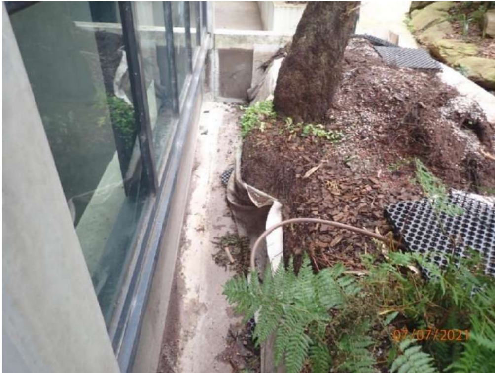
Photograph 81 – Planter box adjacent to staircase 01
