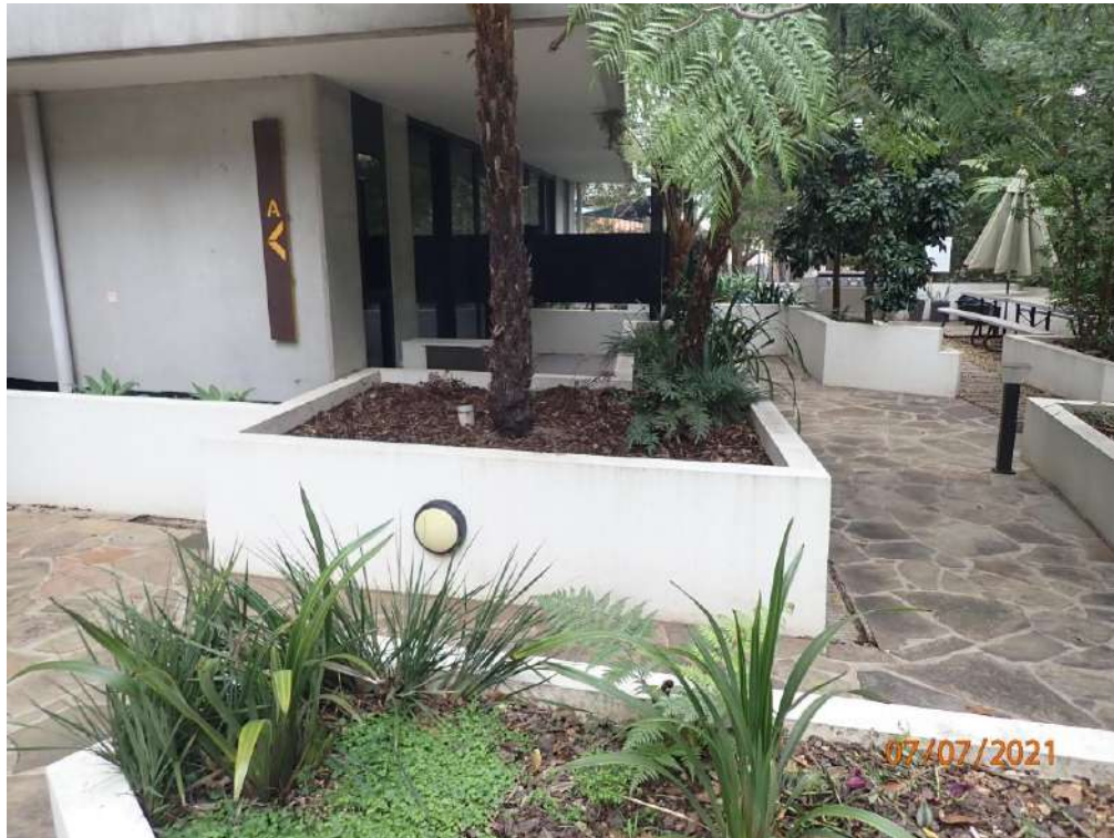
Photograph 77 - Paving directly above basement carpark
