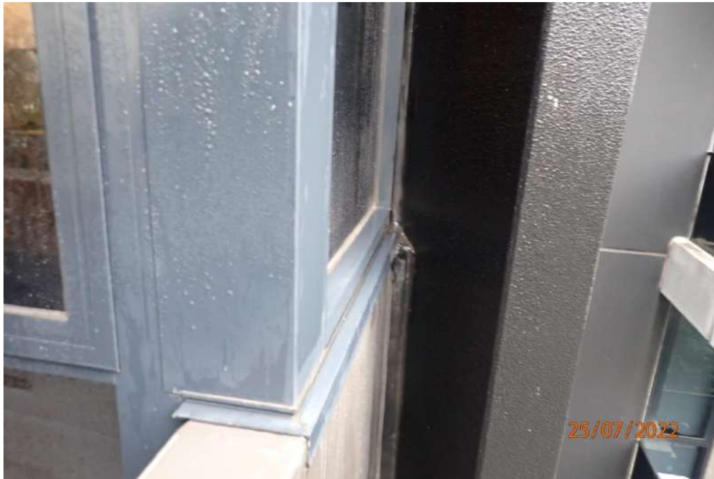
Photograph 183 - Lot 324B/Apartment 336B, water testing to north west apartment windows
