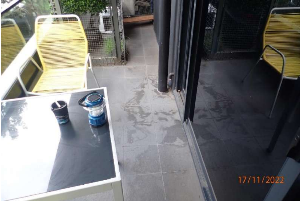
Photograph 105 – Apartment 205A balcony
