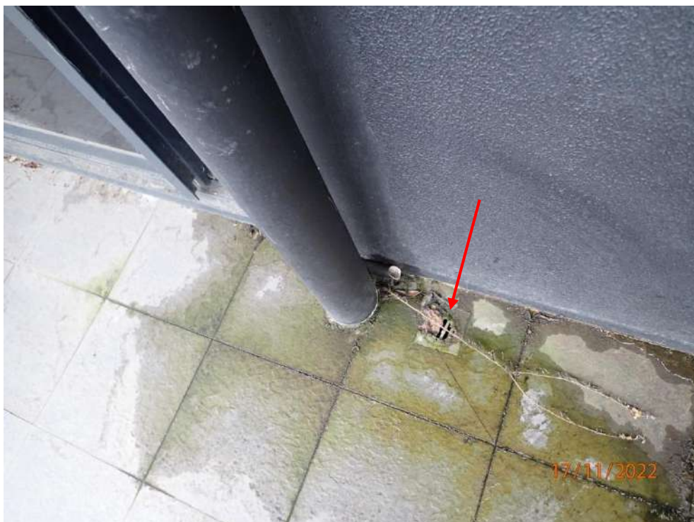
Photograph 18 - Apartment 308A balcony drainage outlet
