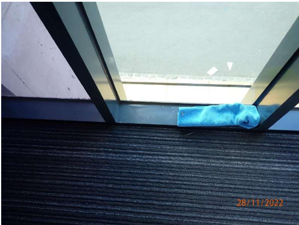
Photograph 82 - Level 4 south passageway aluminium windows
