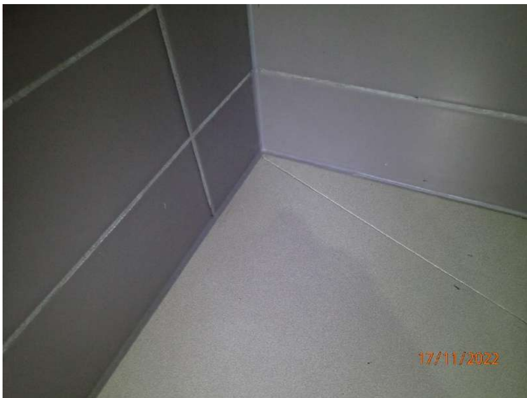
Photograph 44 - Apartment 328B bathroom shower, new flexible sealant to floor perimeter
