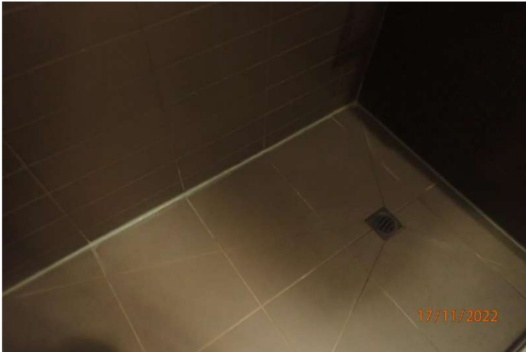
Photograph 123 - Apartment 521B bathroom shower, resealing of tiled floor perimeter
