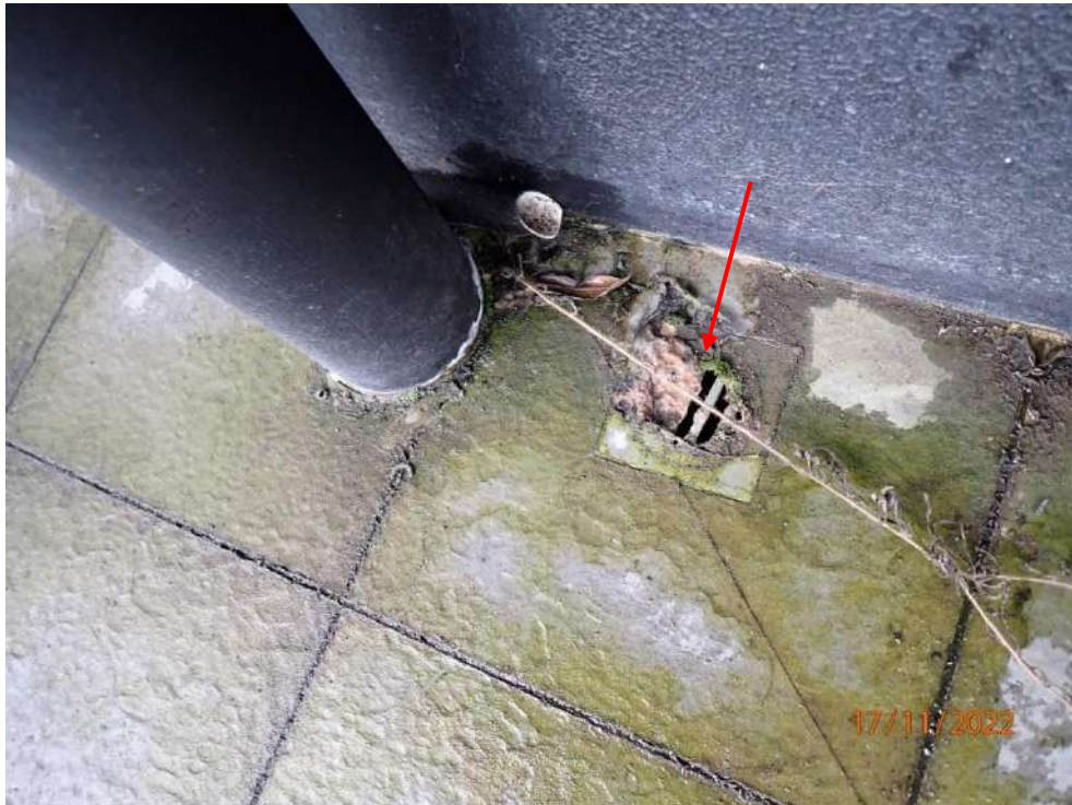
Photograph 19 - Apartment 308A balcony drainage outlet
