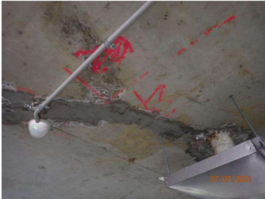
Photograph 55 – Cracking repairs to concrete of basement ceiling
