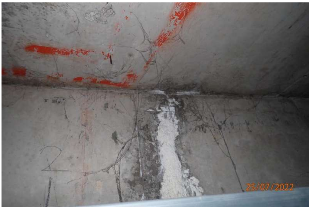
Photograph 154 - Upper basement level, beneath Lot 110A/Apartment 110A planter boxes
