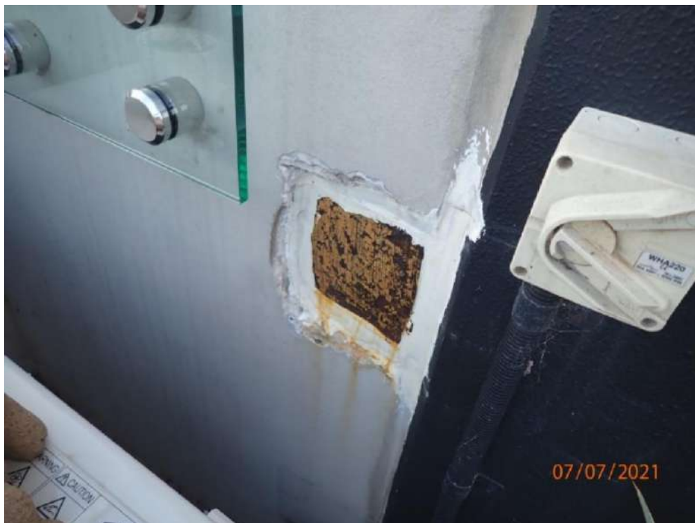
Photograph 110 – Tension plates filled with silicone
