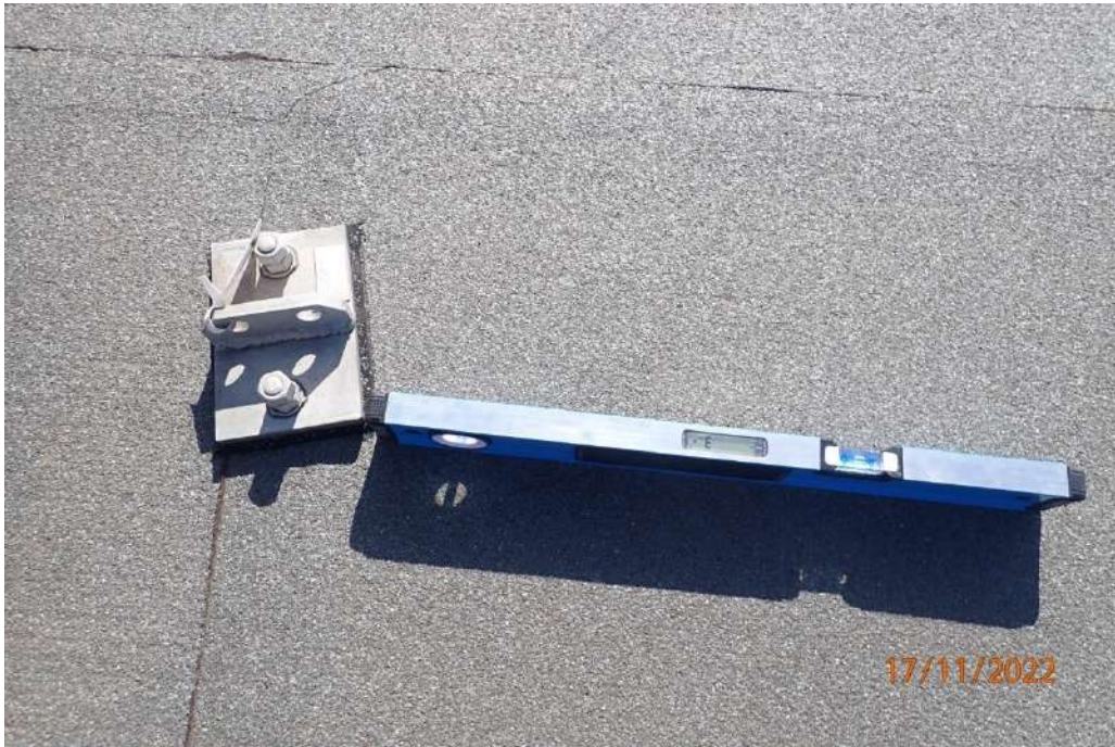
Photograph 139 - Rooftop above Apartment 510A bedroom, anchor point
