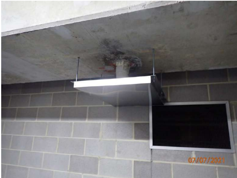
Photograph 5 – Builder installed tray below PVC pipe above carpark 70
