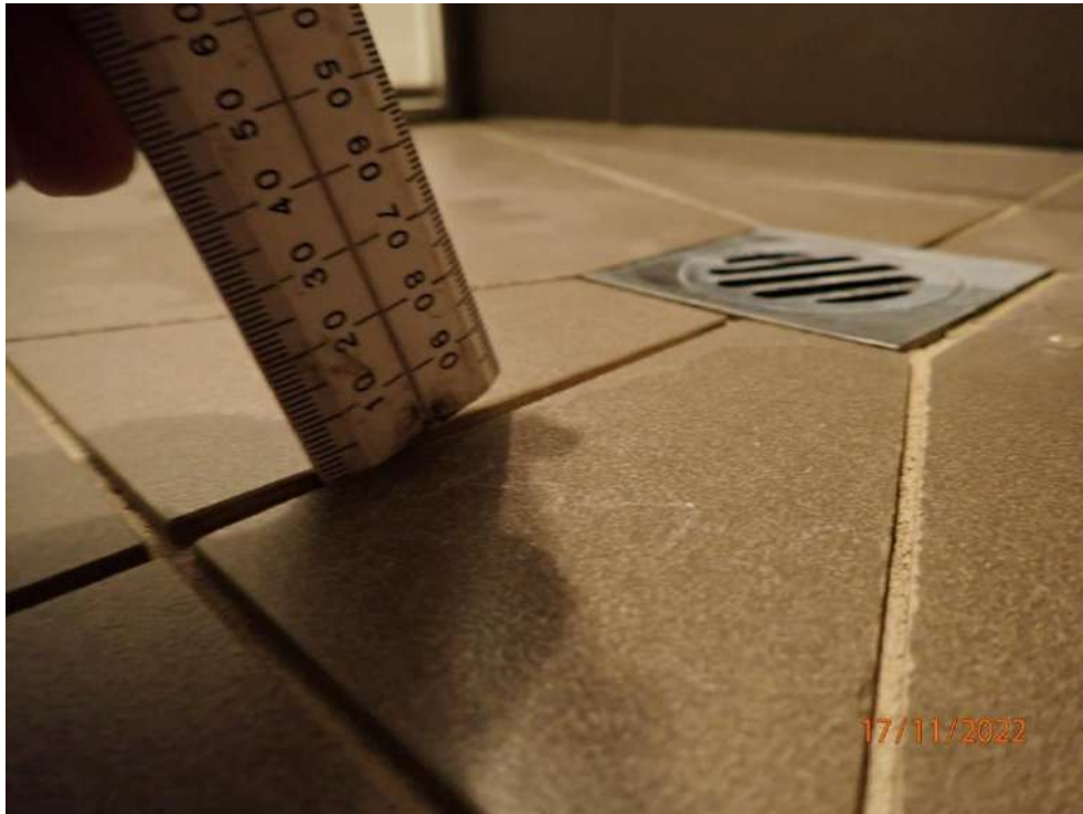
Photograph 9 - Apartment 309A bathroom shower recessed grout lines
