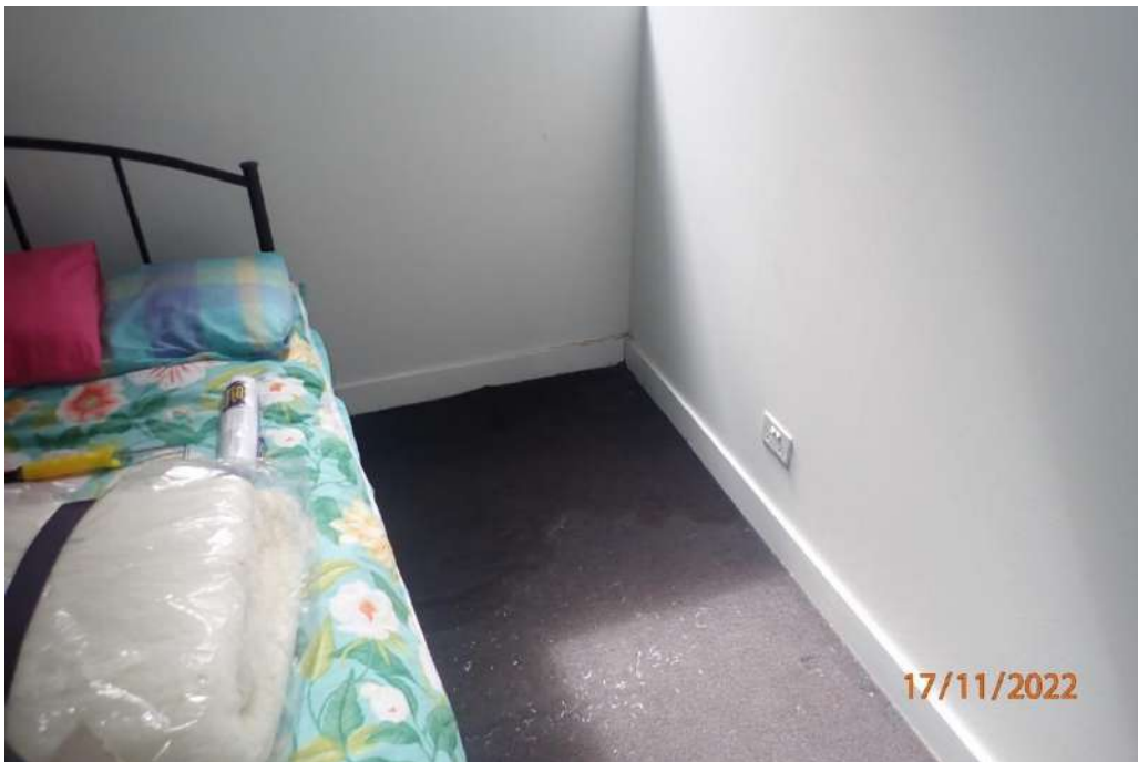
Photograph 110 – Apartment 126B, southeast corner of bedroom 2
