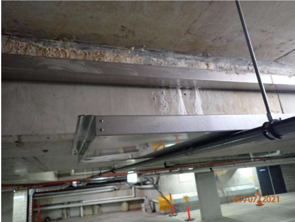
Photograph 51 - Drip tray installed to basement carpark below areas of efflorescence and calcium build up
