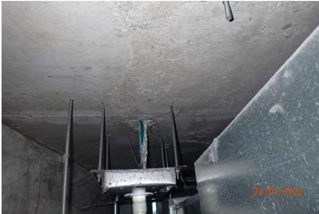
Photograph 155 - Upper basement level, beneath Lot 110A/Apartment 110A planter boxes
