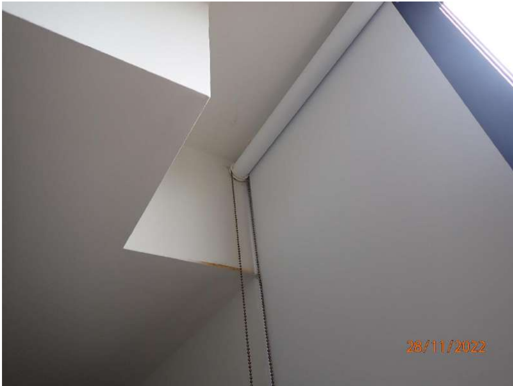
Photograph 99 – Apartment 604B, living area opening pelmet
