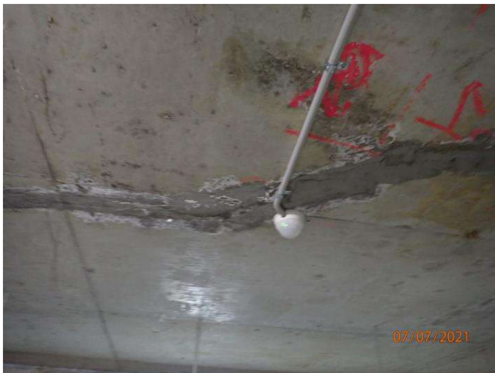
Photograph 54 – Cracking repairs to concrete of basement ceiling
