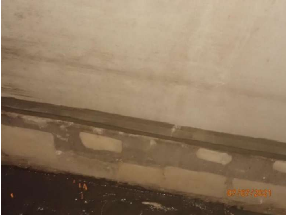
Photograph 91 – Waterproofing and sealant applied to water tank
