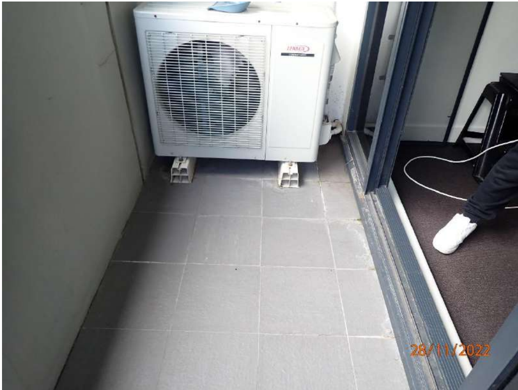
Photograph 87 – Apartment 431B balcony
