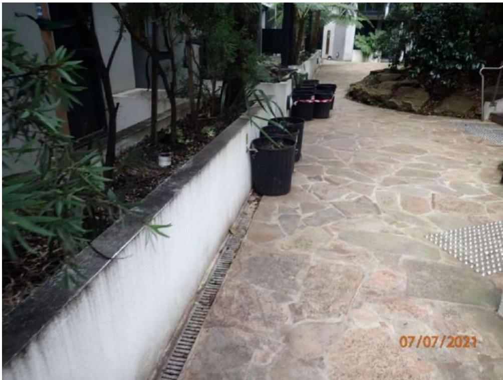
Photograph 76 - Paving directly above basement carpark
