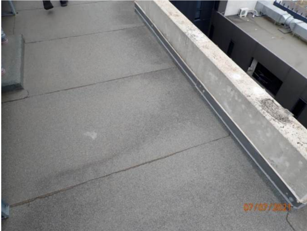
Photograph 133 - Pressure flashings to Butynol sheets fixed to concrete wall at more than 750 mm centres to roofing of buildings A and B
