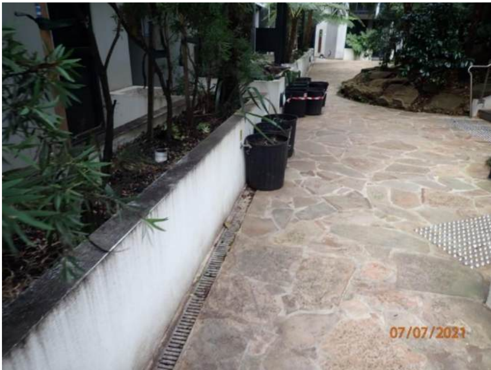
Photograph 76 - Paving directly above basement carpark
