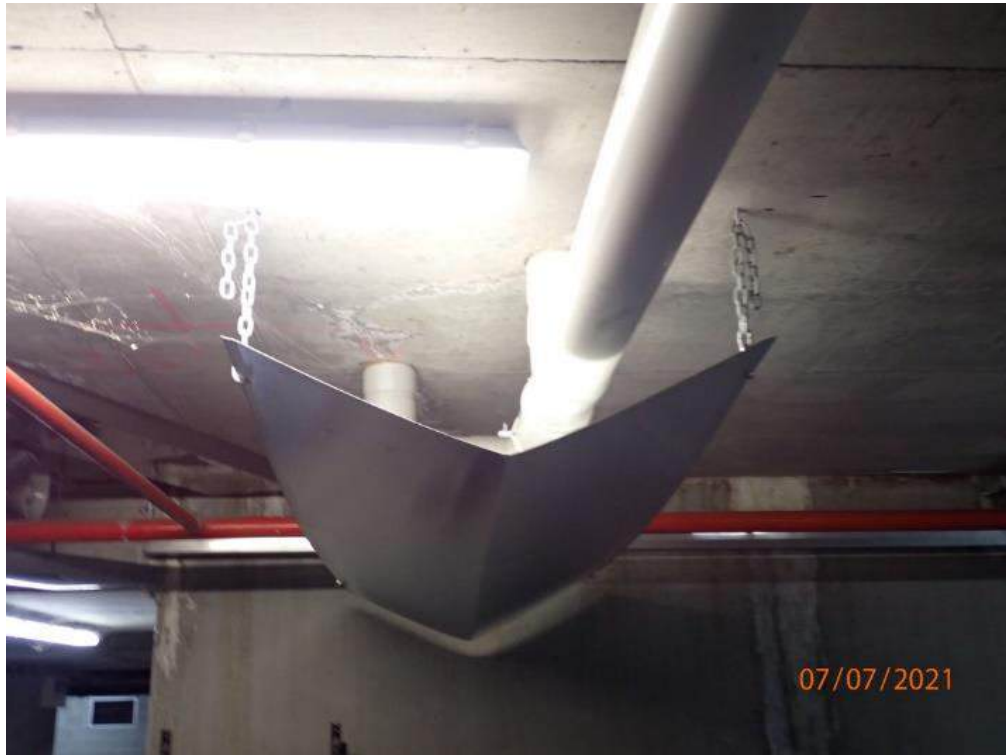
Photograph 57 – Drip tray installed below pipe penetration
