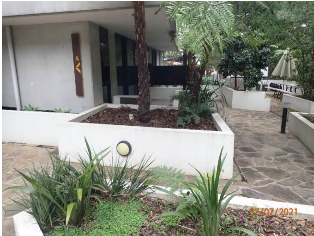
Photograph 77 - Paving directly above basement carpark
