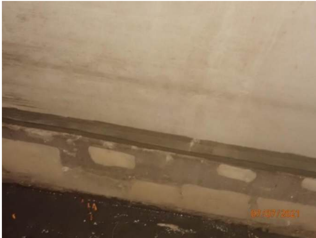
Photograph 91 – Waterproofing and sealant applied to water tank
