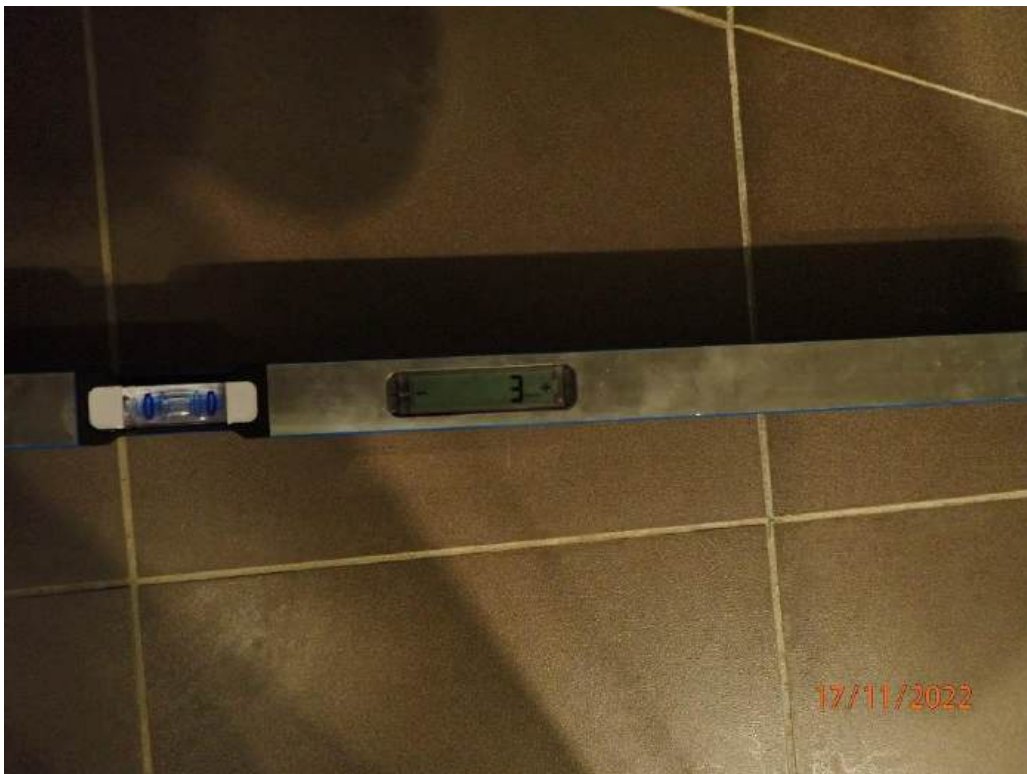
Photograph 28 - Apartment 526B bathroom shower fall 1 in 333
