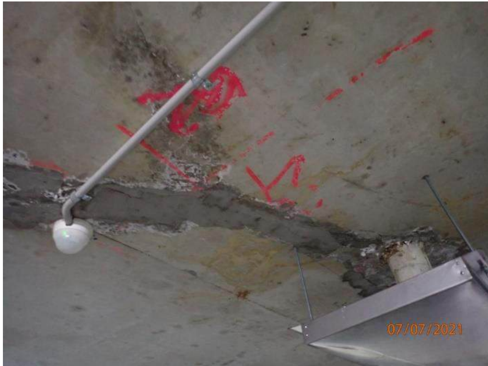
Photograph 55 – Cracking repairs to concrete of basement ceiling
