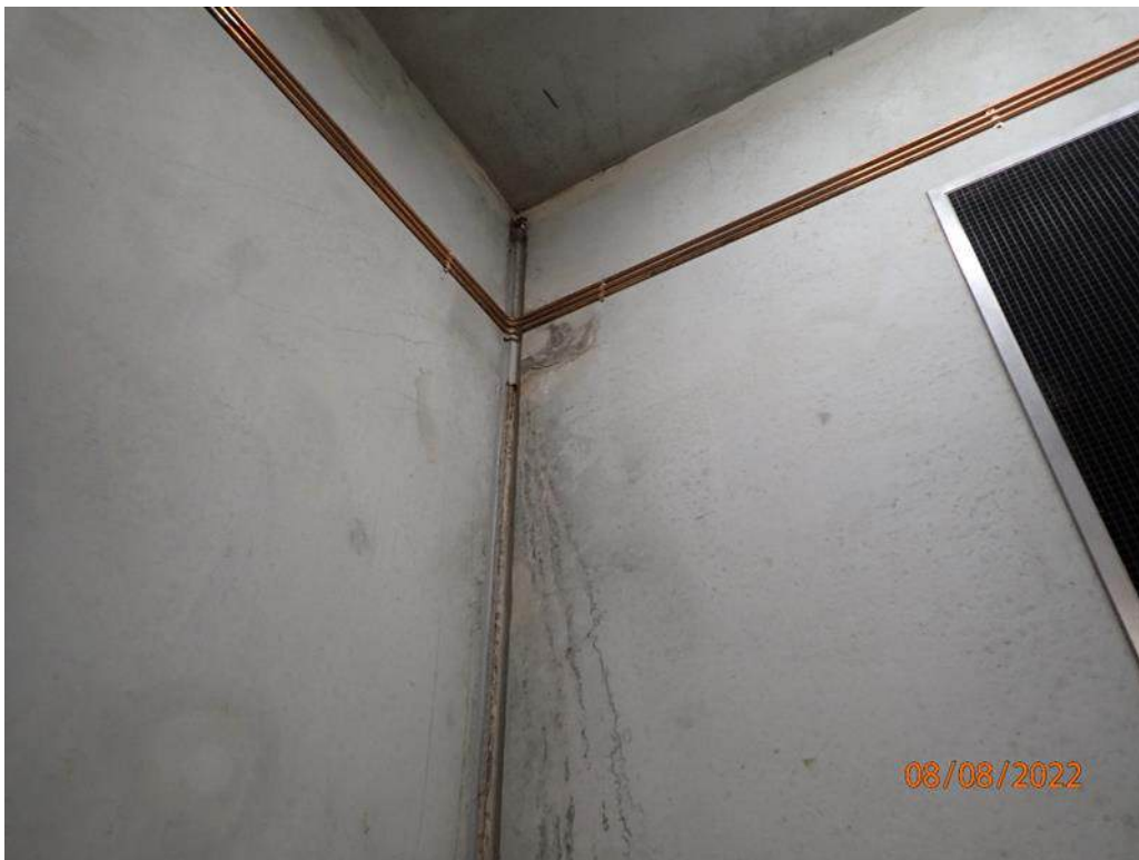
Photograph 138 - Building B north west corner of the north stairwell wall at rooftop level
