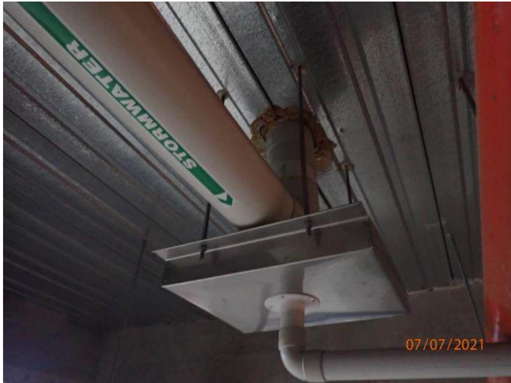
Photograph 43 – Drip tray installed below pipe penetration
