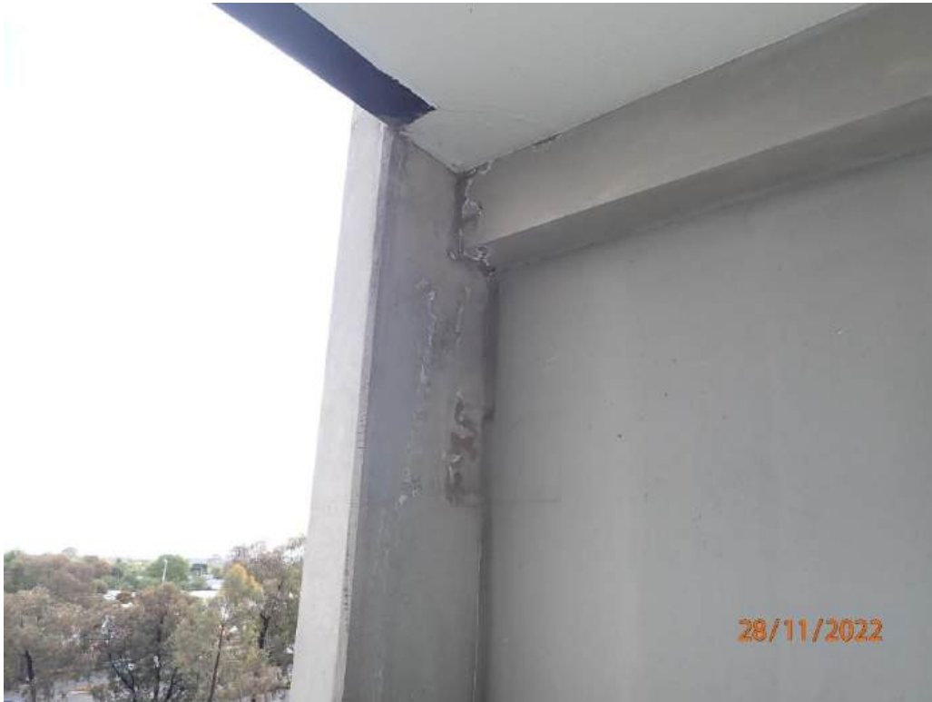
Photograph 75 – Apartment 518B, northeast balcony wall
