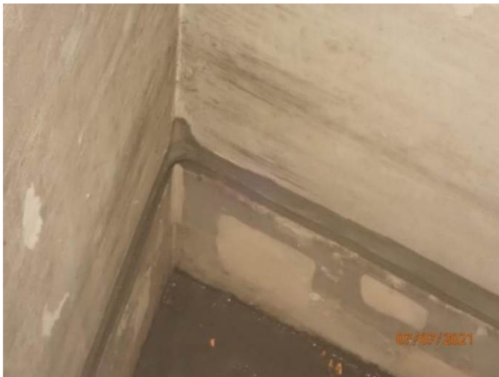
Photograph 90 – Waterproofing and sealant applied to water tank
