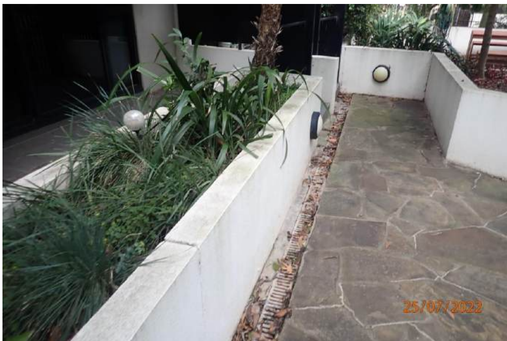
Photograph 152 - Lot 110A/Apartment 110A, courtyard planter box facing west
