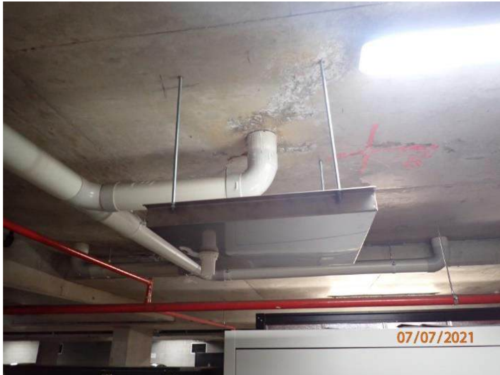
Photograph 39 – Drip tray installed below pipe penetration
