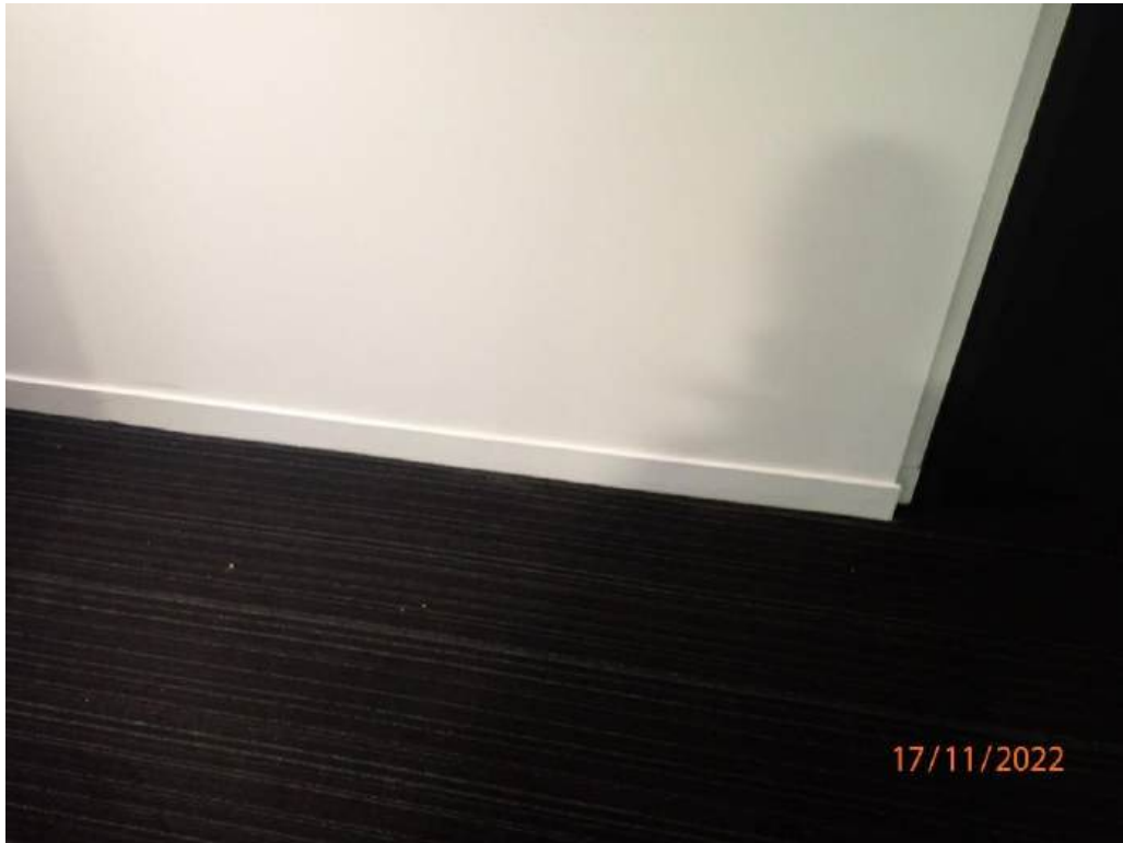
Photograph 41 – Common passageway outside Apartment 328B
