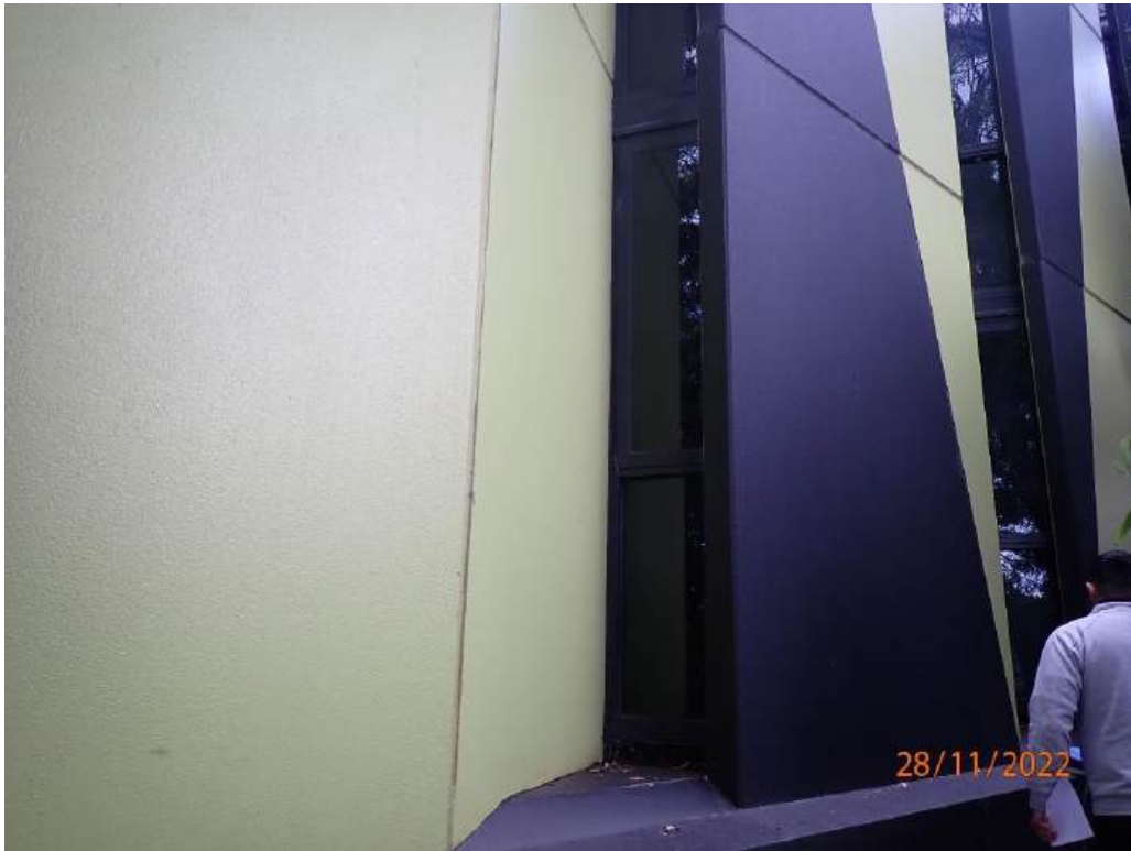
Photograph 71 - Apartment 109A, water testing to bedroom 2 west window
