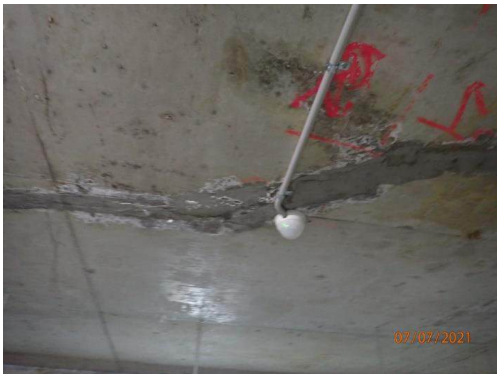
Photograph 54 – Cracking repairs to concrete of basement ceiling
