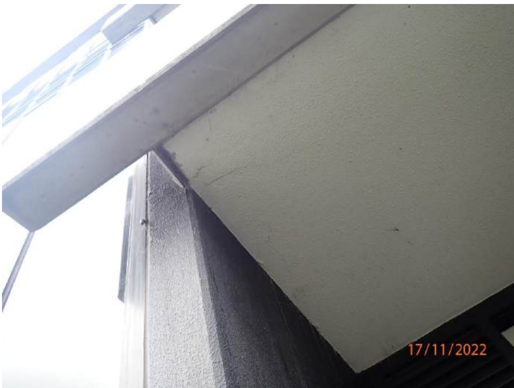
Photograph 24 - Apartment 308A balcony west wall
