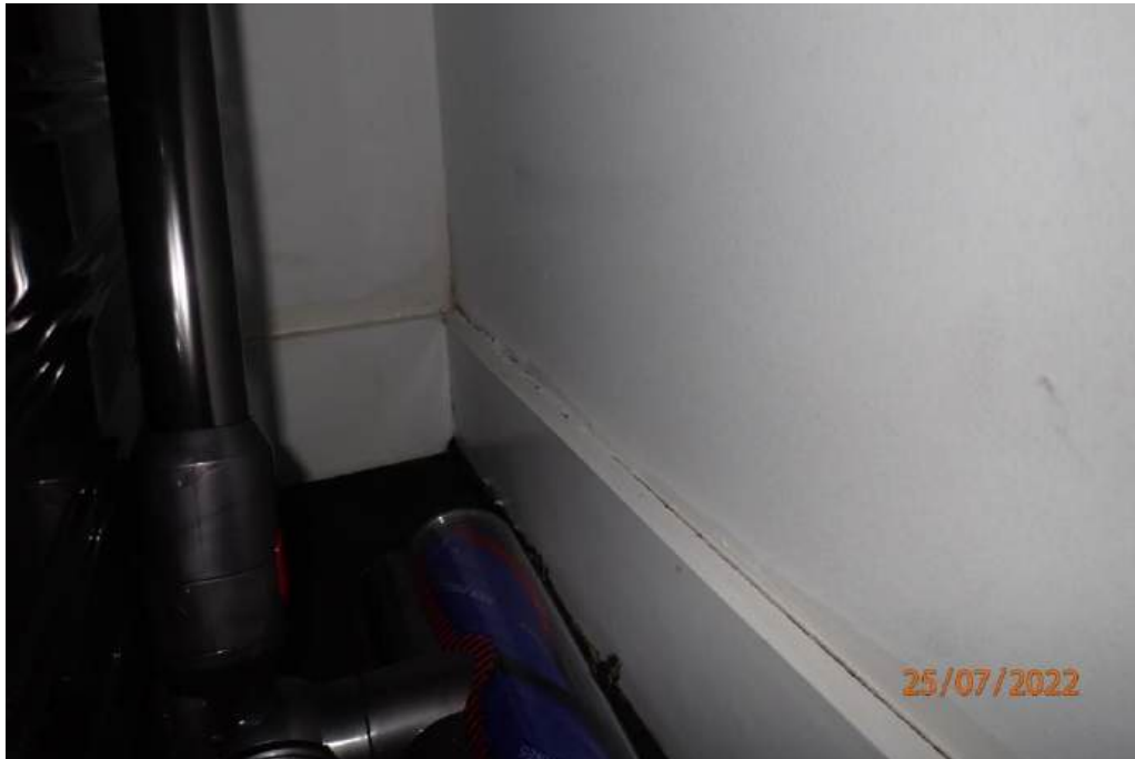
Photograph 143 - Lot 106B/Apartment 116B, southwest corner of bedroom skirting trim
