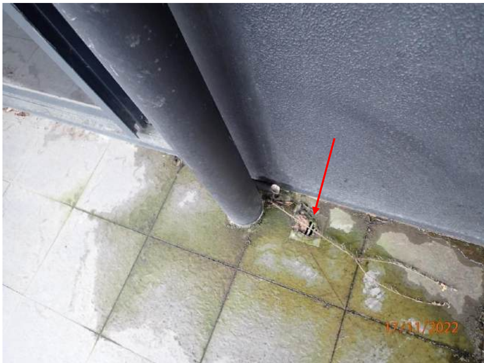
Photograph 18 - Apartment 308A balcony drainage outlet
