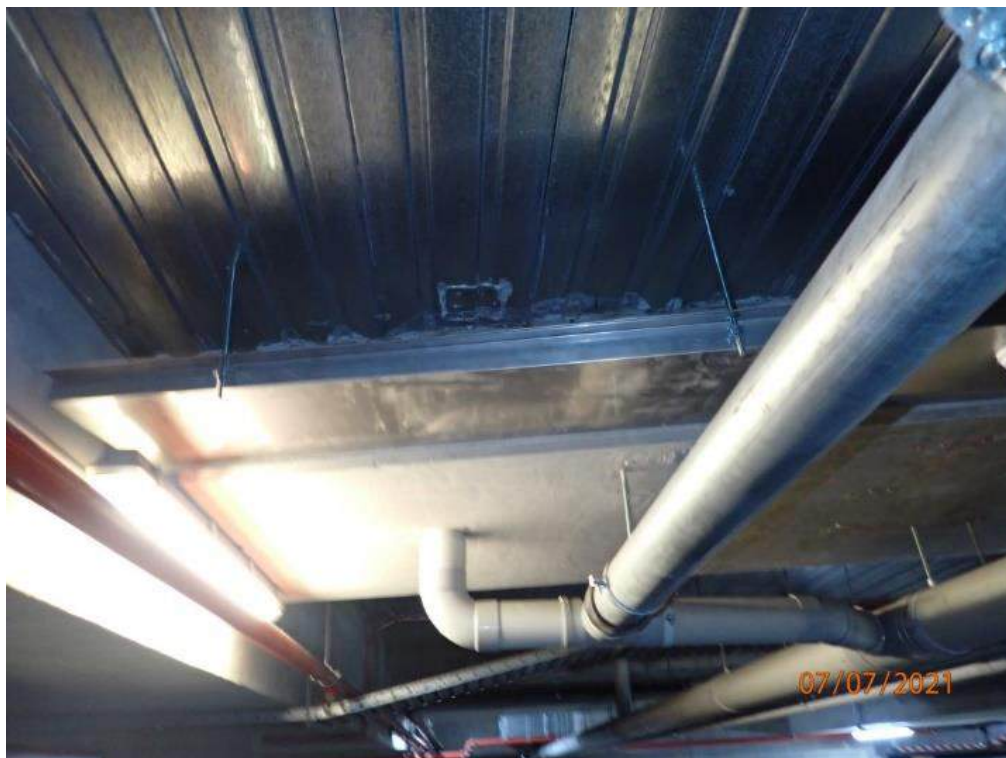
Photograph 44 - Drip tray installed below areas of efflorescence
