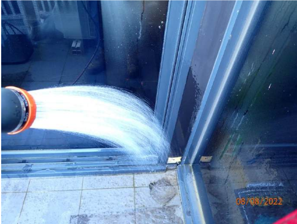
Photograph 215 - 704B/Apartment 703B, water testing to living sliding door opening to balcony
