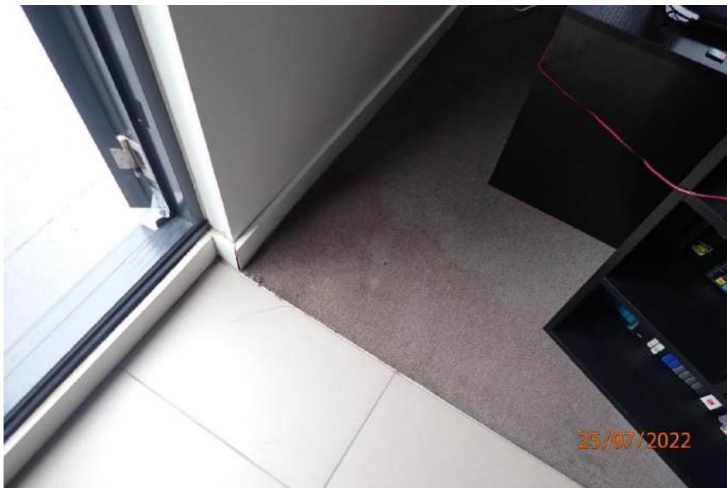
Photograph 194 - Lot 607B/Apartment 605B, west wall opening to the balcony
