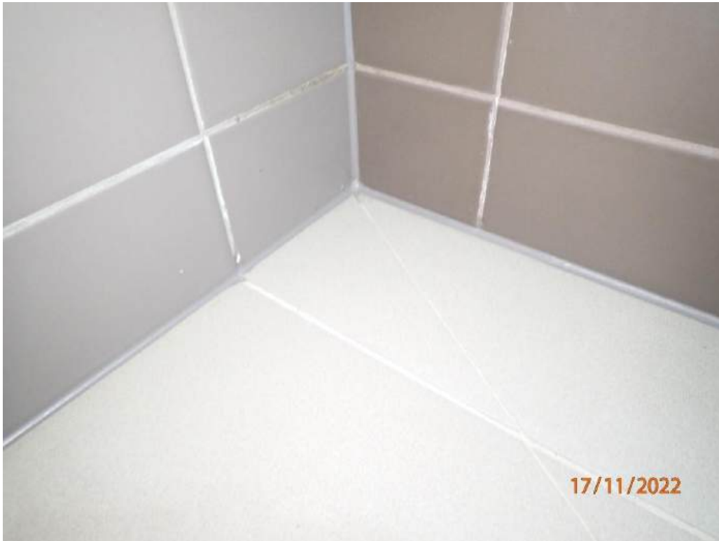
Photograph 45 - Apartment 328B bathroom shower, new flexible sealant to floor perimeter
