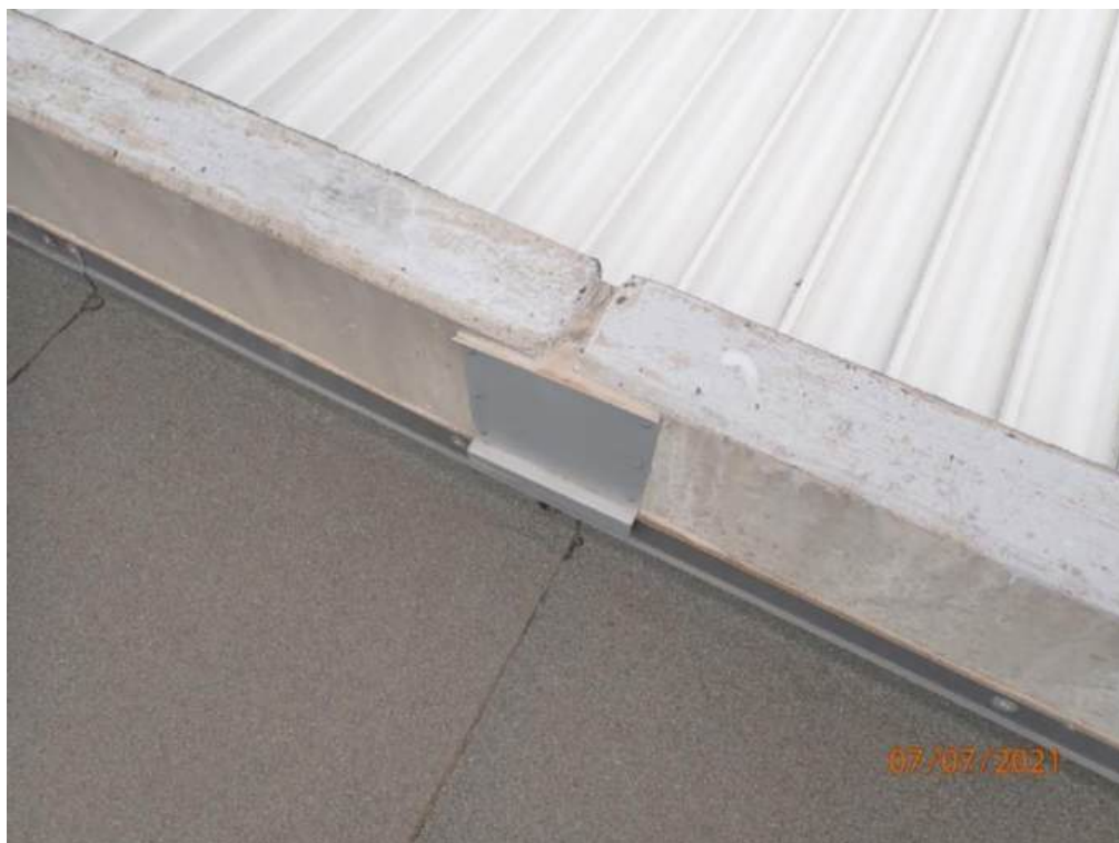
Photograph 122 – Metal plates fixed to large gaps between concrete wall panels on building B roof
