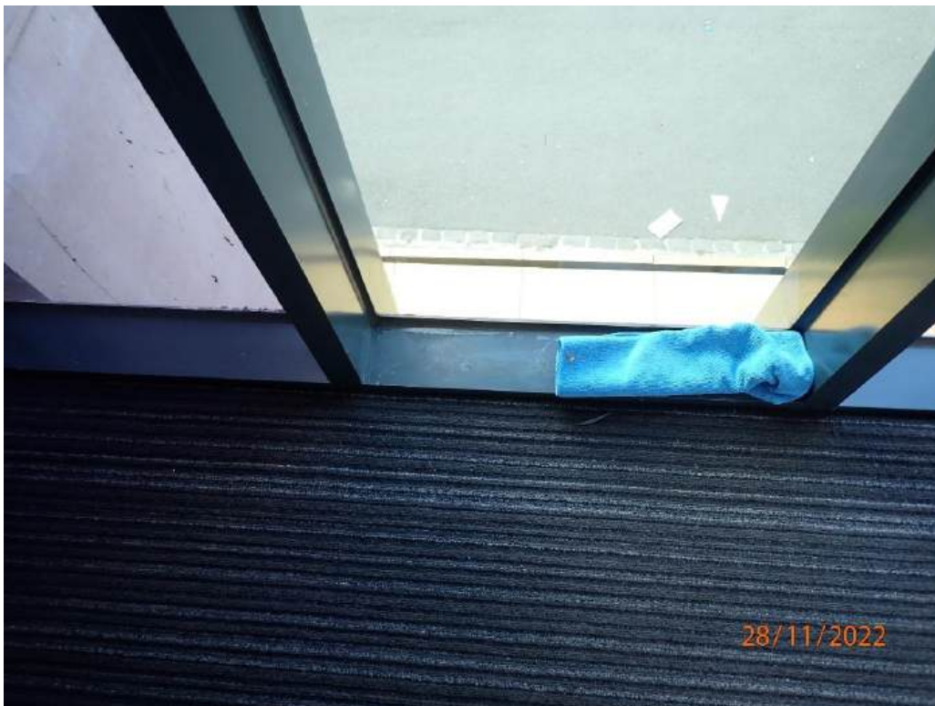
Photograph 82 - Level 4 south passageway aluminium windows
