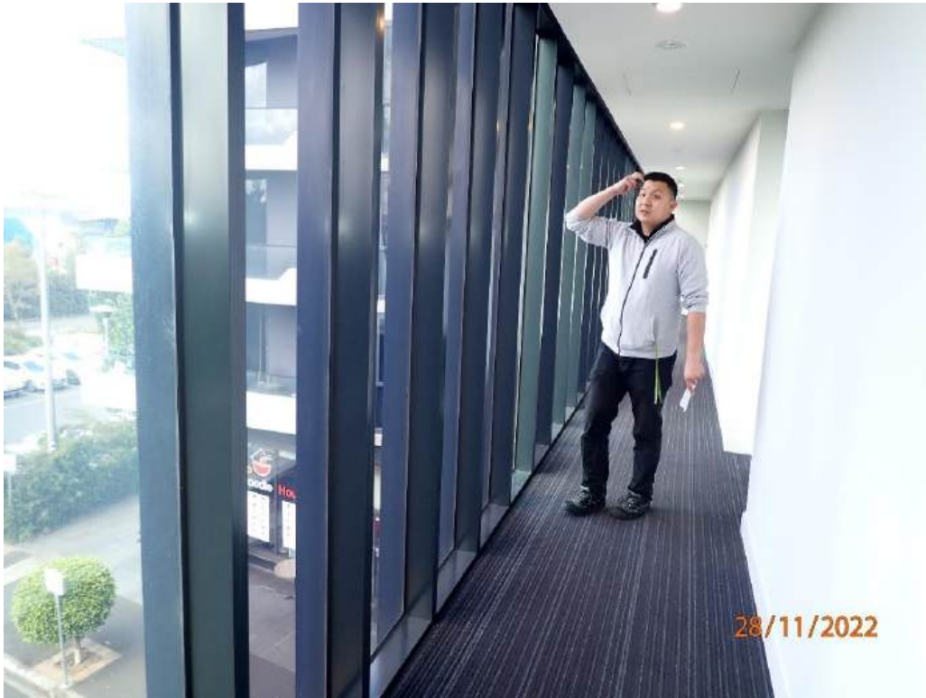
Photograph 81 – Level 4 south passageway aluminium windows
