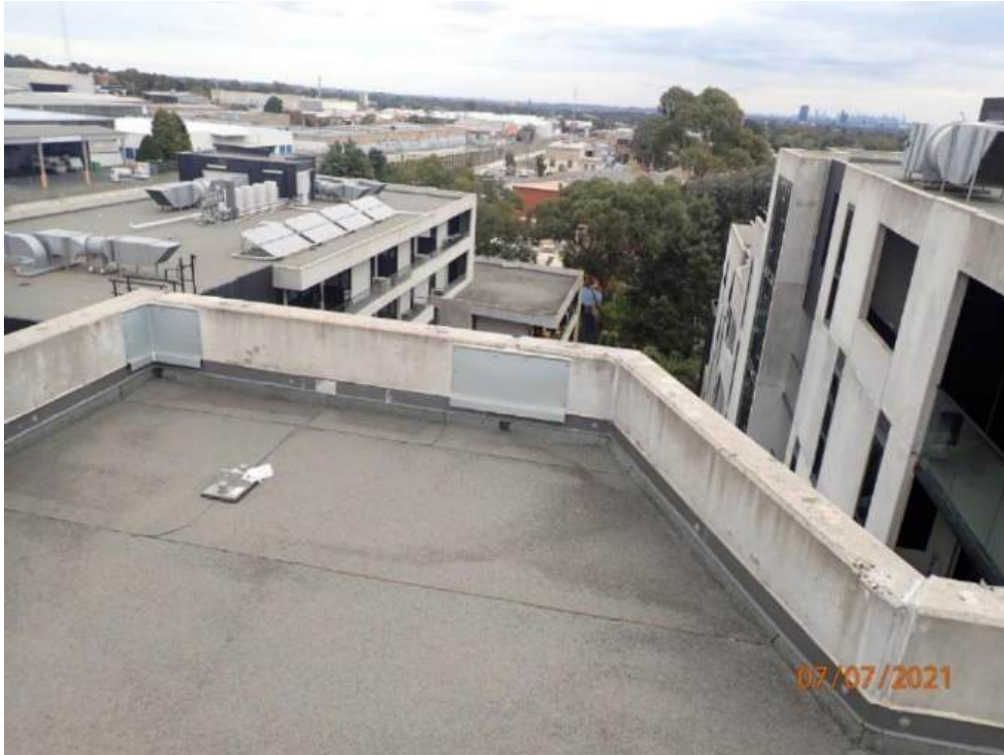
Photograph 119 – Metal plates fixed to large gaps between concrete wall panels on building B roof
