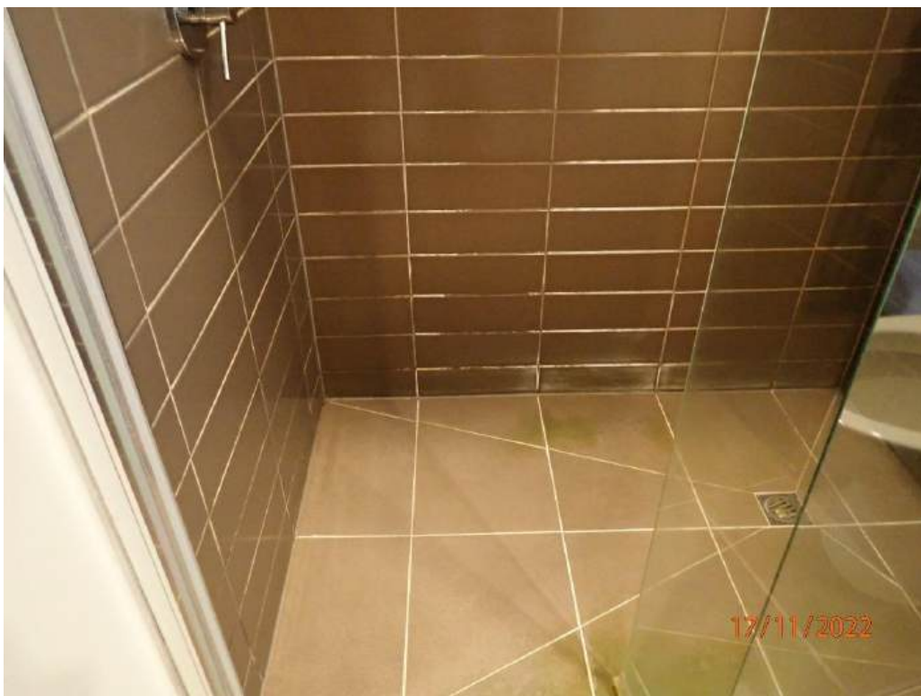
Photograph 26 – Apartment 526B bathroom shower
