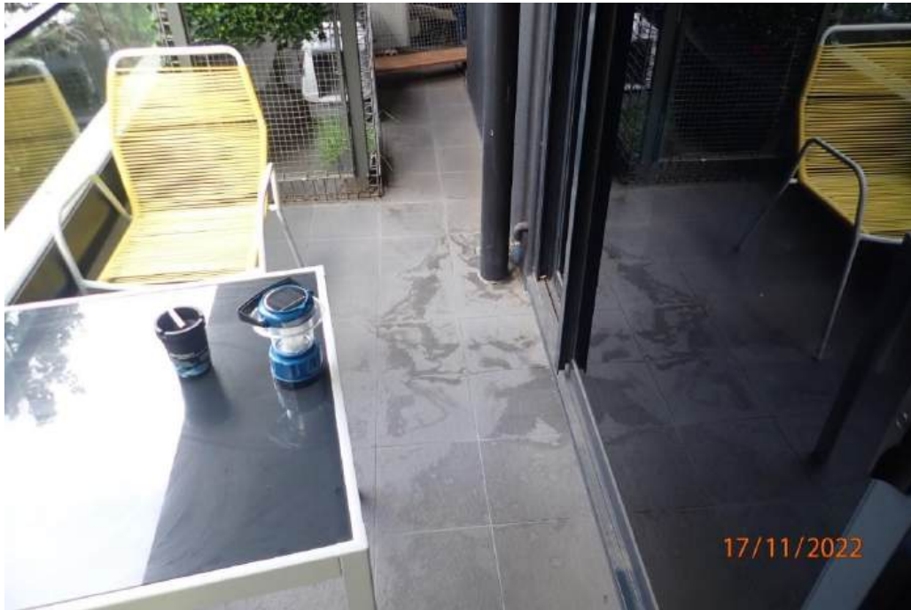
Photograph 105 – Apartment 205A balcony
