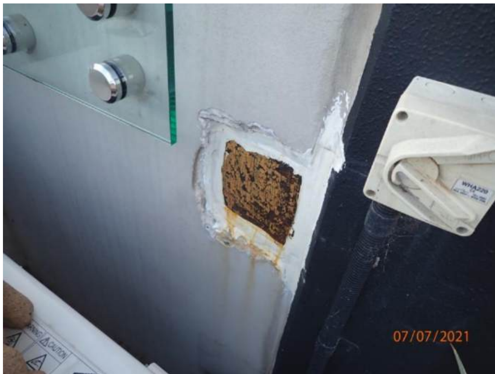
Photograph 110 – Tension plates filled with silicone
