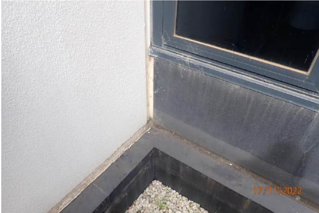
Photograph 111 - Apartment 126B, external view of window, southeast corner of bedroom 2
