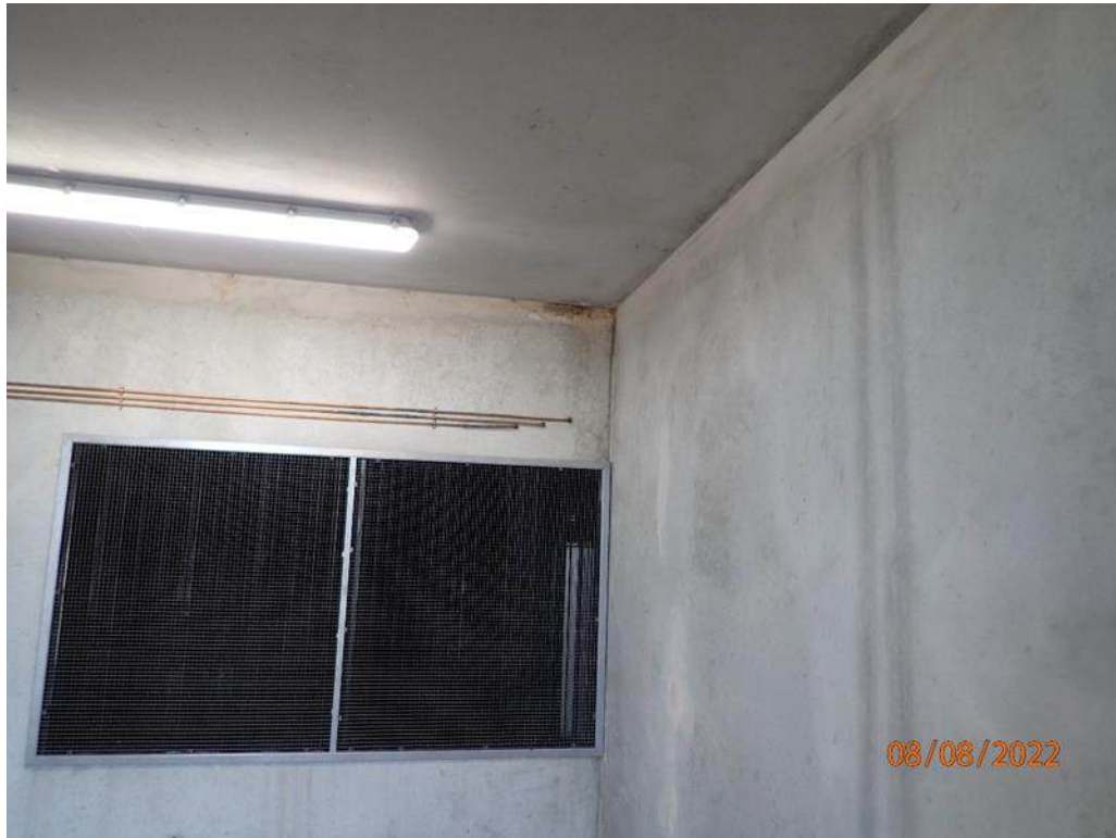
Photograph 139 - Building B north east corner of the north stairwell wall at rooftop level
