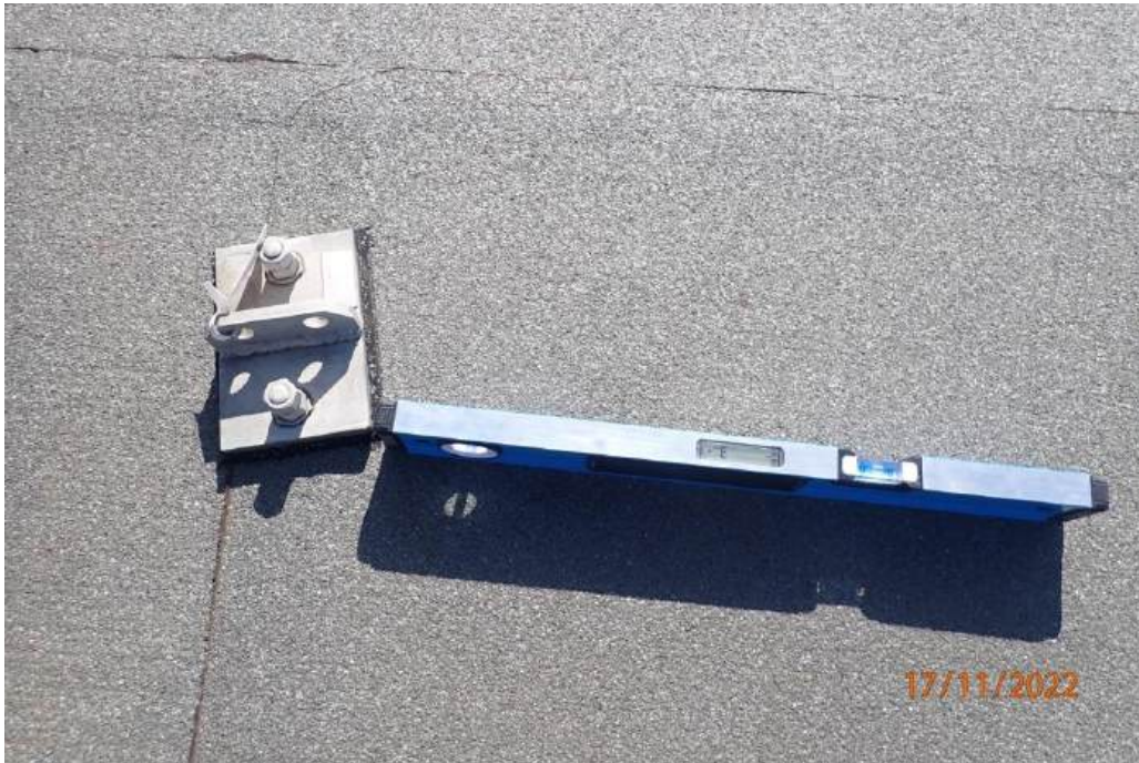
Photograph 139 - Rooftop above Apartment 510A bedroom, anchor point
