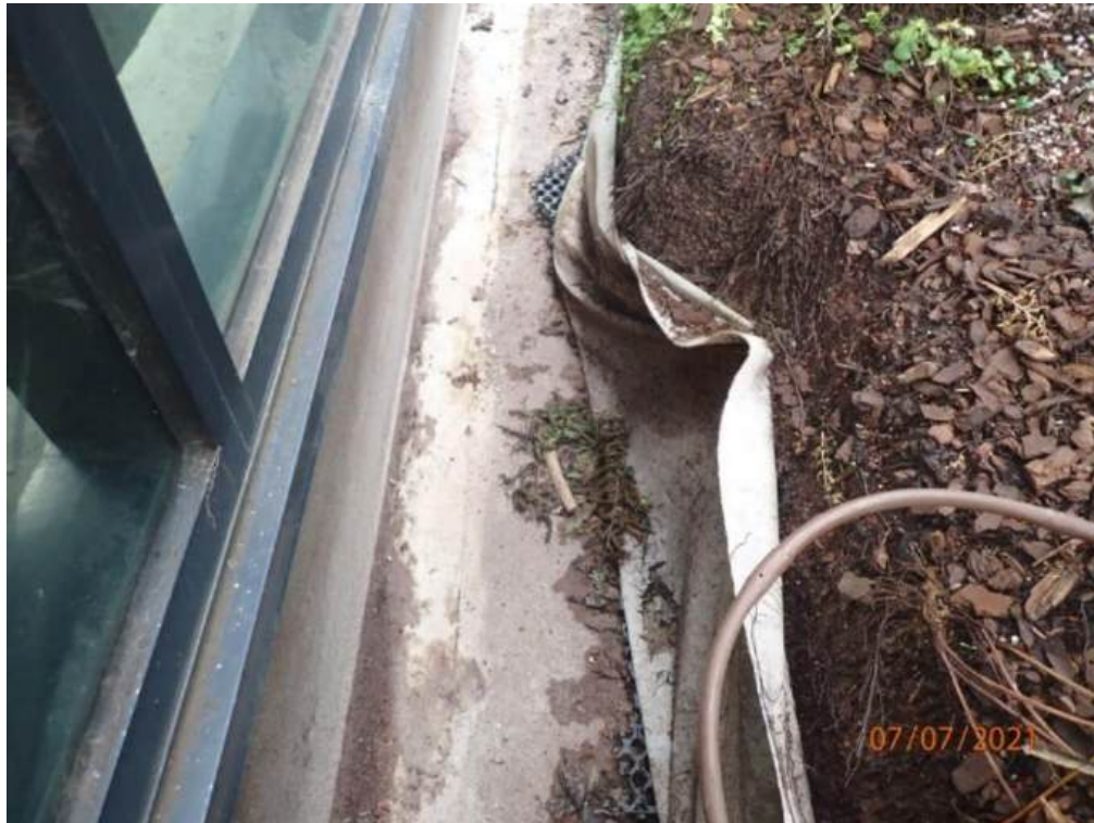
Photograph 83 – Internal waterproof membrane to planter box
