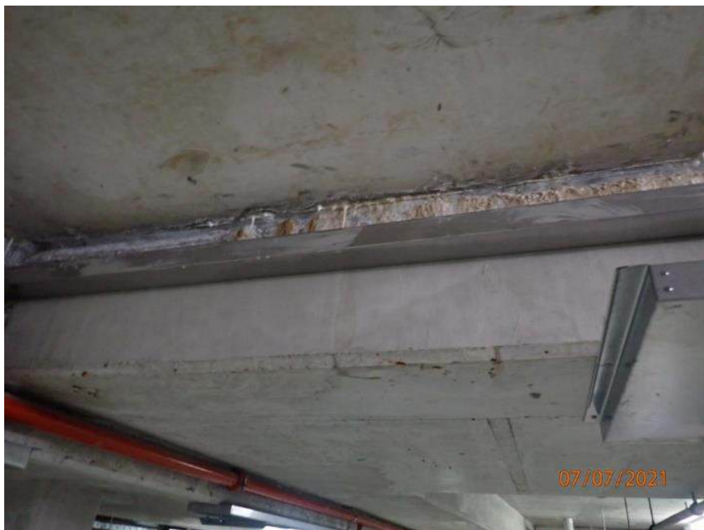
Photograph 52 - Drip tray installed to basement carpark below areas of efflorescence and calcium build up
