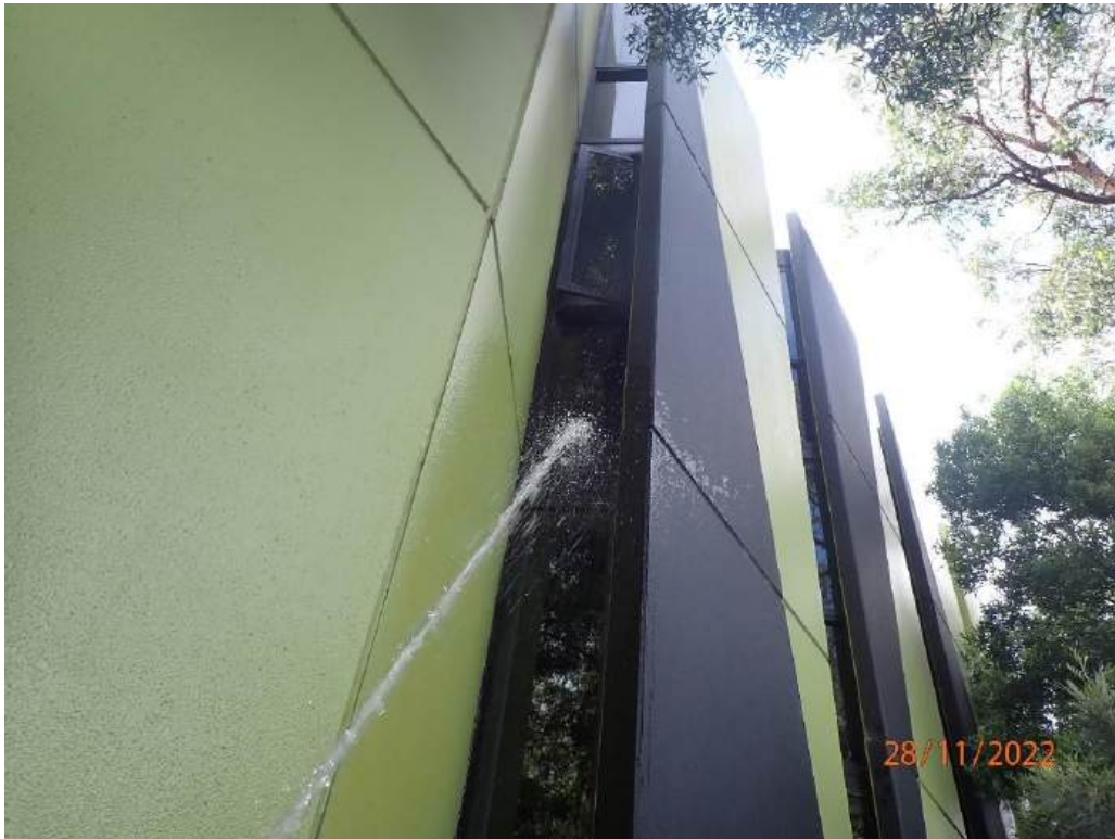
Photograph 73 - Apartment 109A, water testing to bedroom 2 west window
