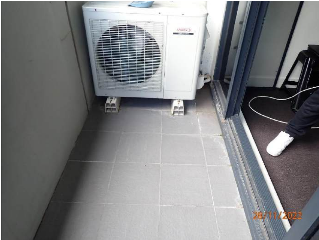
Photograph 87 – Apartment 431B balcony
