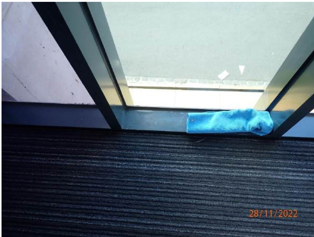
Photograph 82 - Level 4 south passageway aluminium windows
