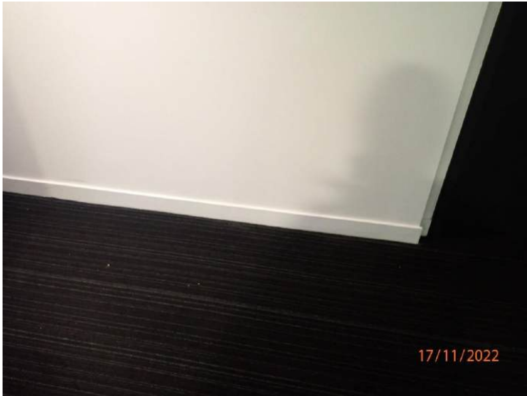
Photograph 41 – Common passageway outside Apartment 328B
