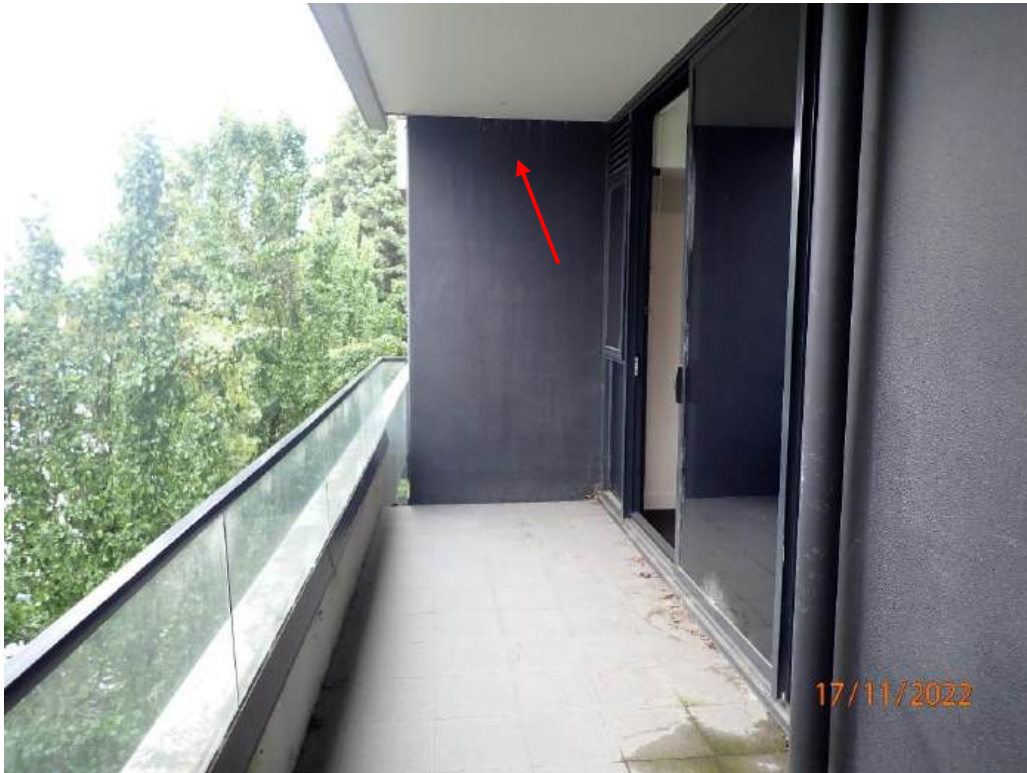
Photograph 21 - Apartment 308A balcony west wall
