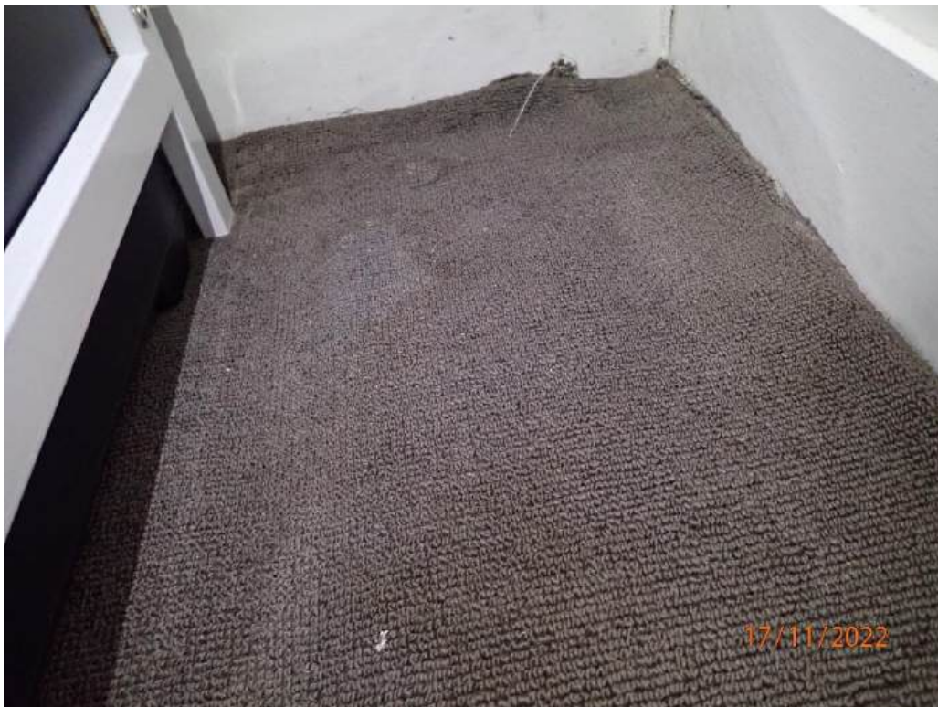
Photograph 60 - Apartment 417B, northwest corner of the living area
