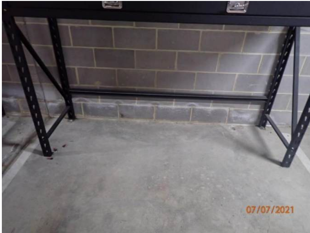
Photograph 89 – Efflorescence to the block walls adjacent the water tanks
