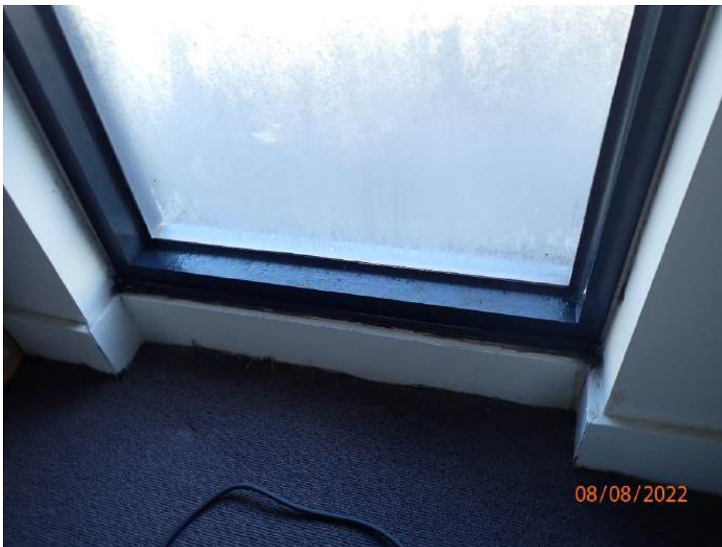
Photograph 202 - 704B/Apartment 703B, west window of the south bedroom
