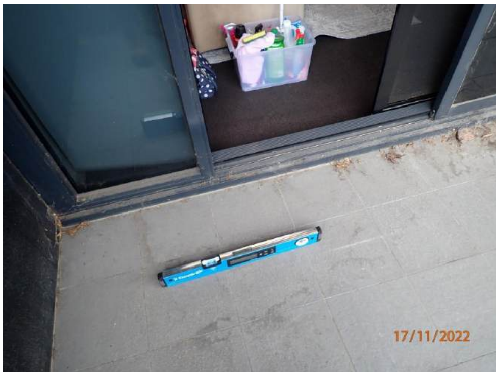
Photograph 10 - Apartment 308A balcony
