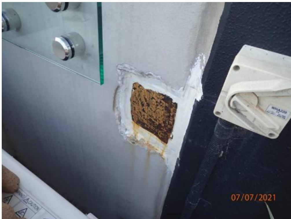
Photograph 110 – Tension plates filled with silicone
