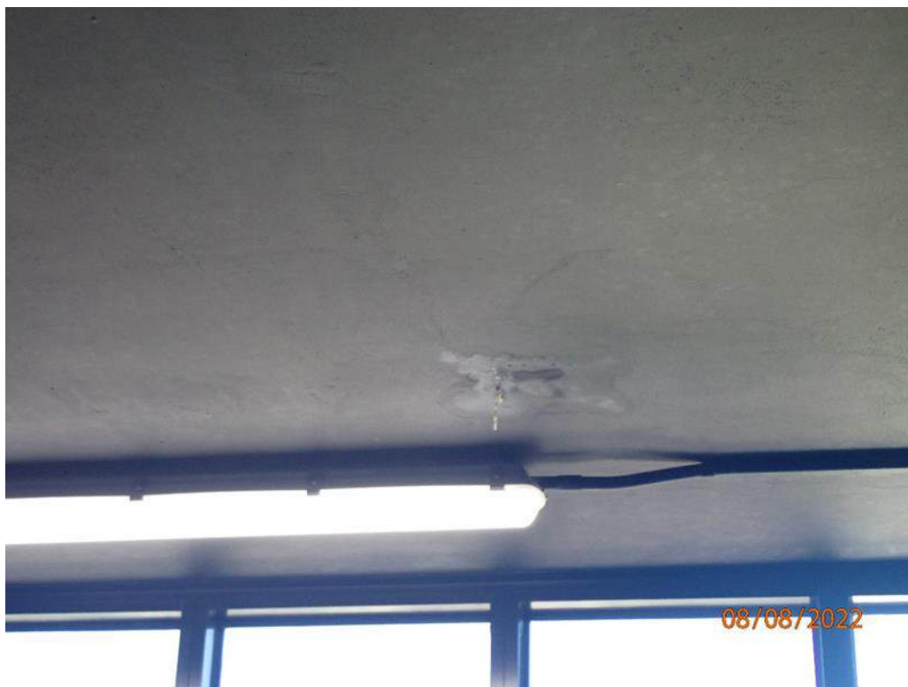
Photograph 136 - Building A centre ceiling of the stairwell at the rooftop level
