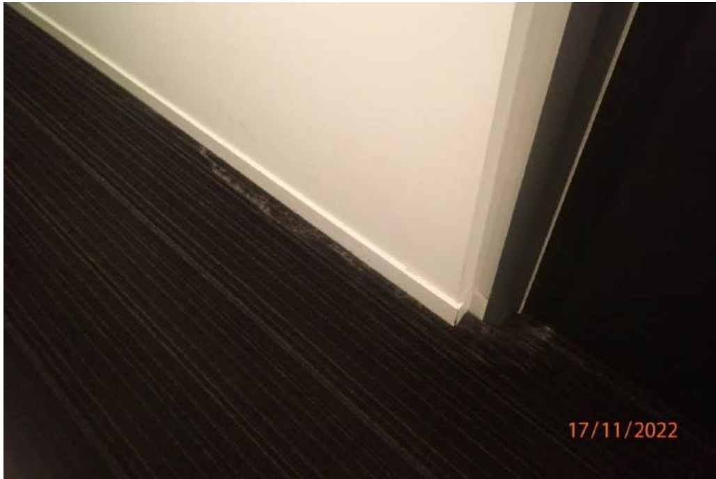
Photograph 117 - Apartment 521B external passageway
