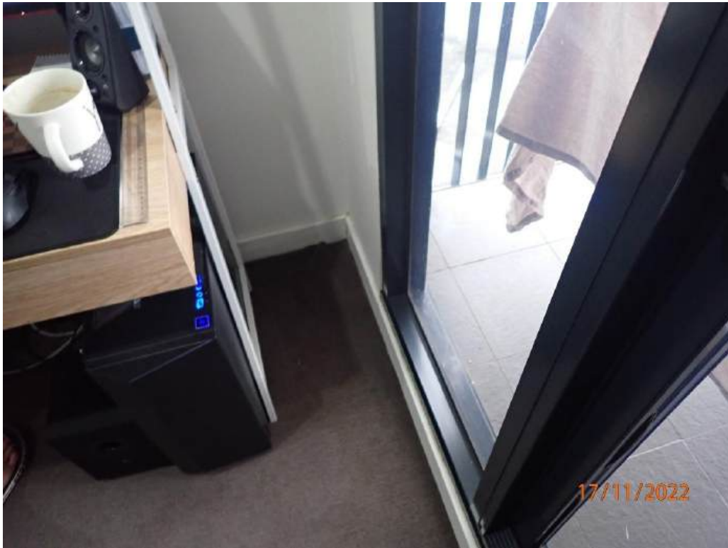
Photograph 59 - Apartment 417B, northwest corner of the living area
