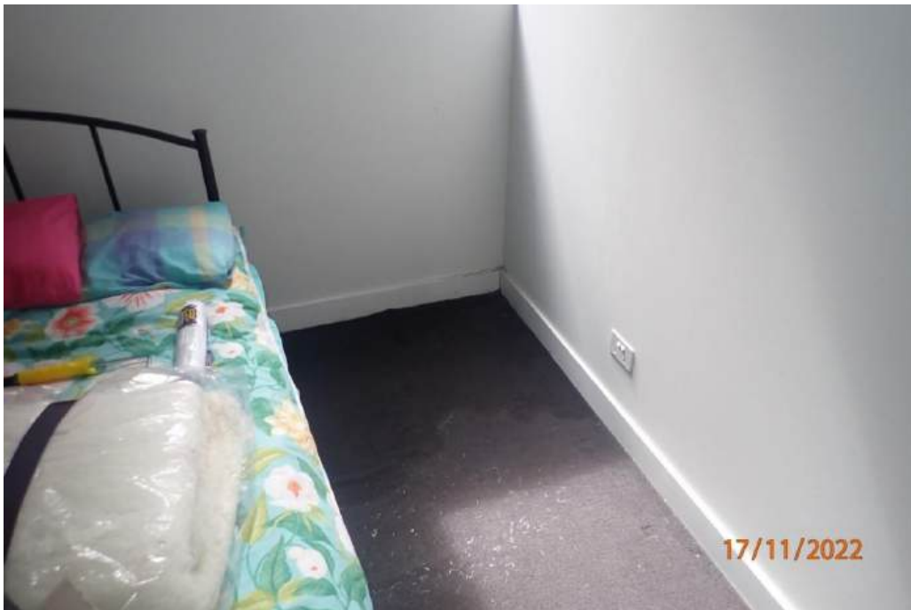
Photograph 110 – Apartment 126B, southeast corner of bedroom 2
