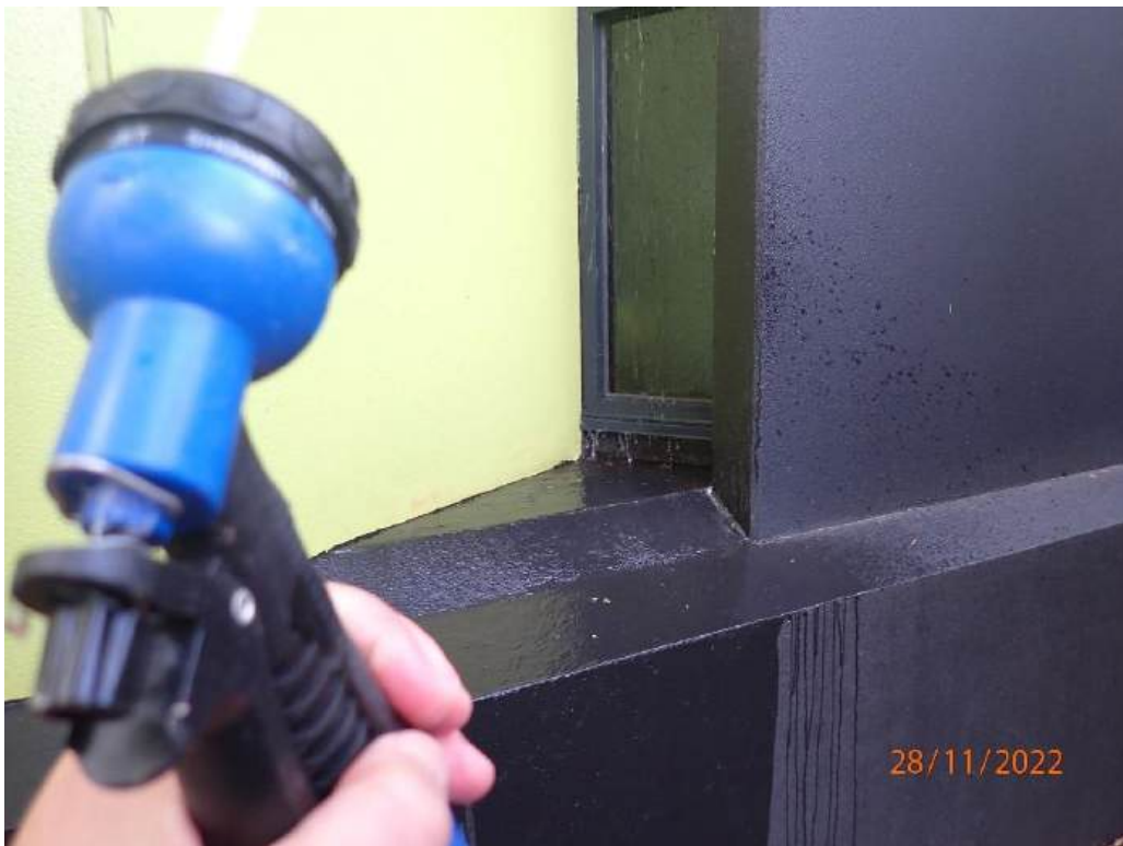
Photograph 72 - Apartment 109A, water testing to bedroom 2 west window
