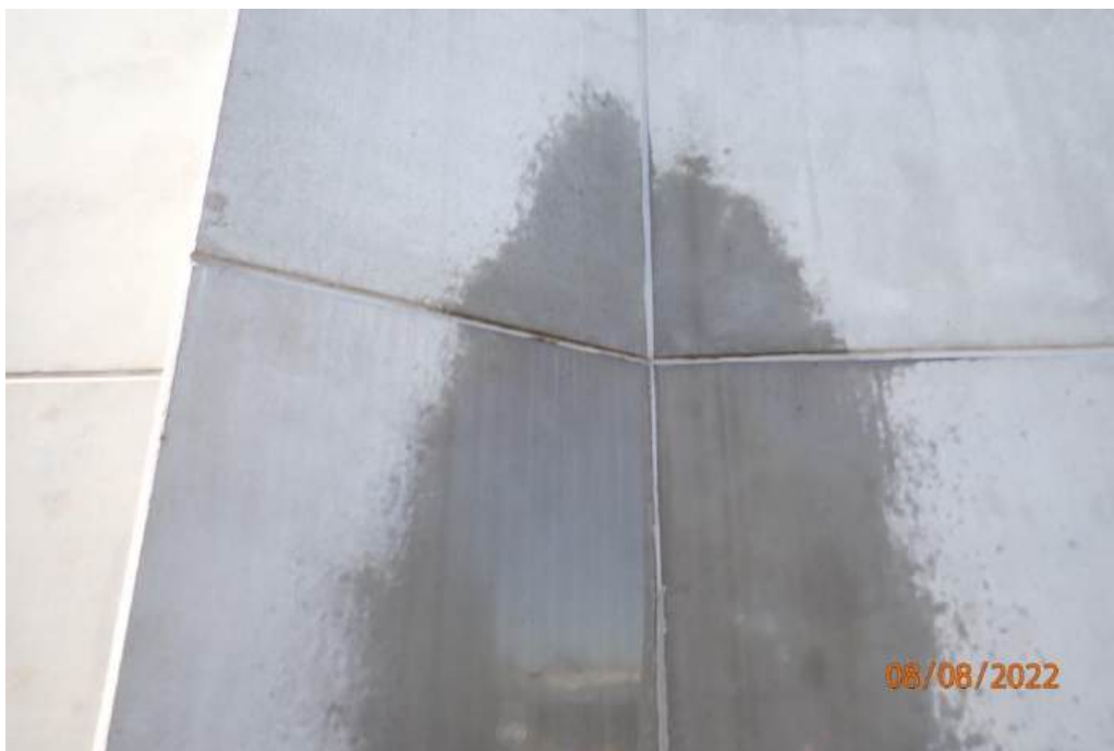
Photograph 188 - Lot 402A/Apartment 402A water testing to west elevation wall
