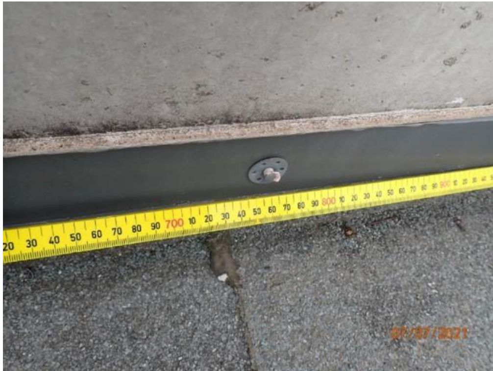
Photograph 131 - Pressure flashings to Butynol sheets fixed to concrete wall at more than 750 mm centres to roofing of buildings A and B
