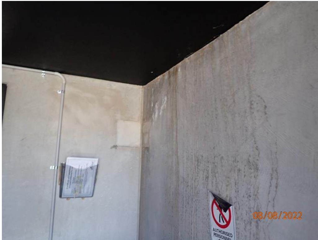
Photograph 135 - Building A north east corner and the centre of the ceiling of the stairwell at the rooftop level
