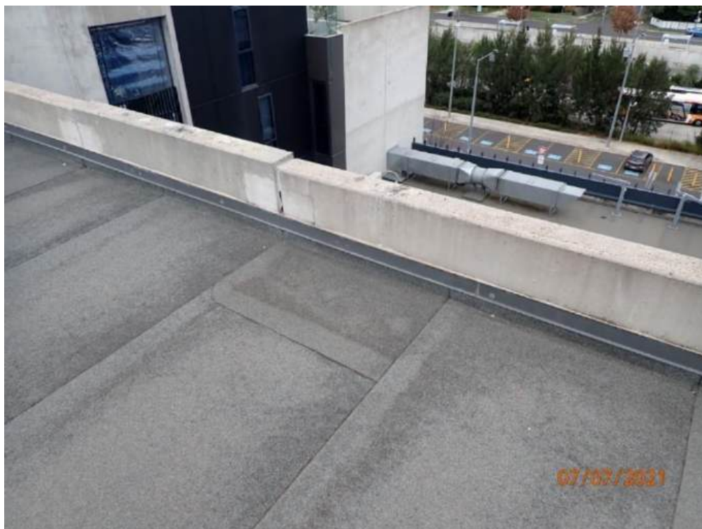
Photograph 132 - Pressure flashings to Butynol sheets fixed to concrete wall at more than 750 mm centres to roofing of buildings A and B
