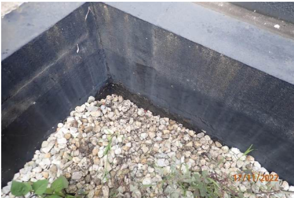
Photograph 112 - Apartment 126B, external view of window and planter box, southeast corner of bedroom 2
