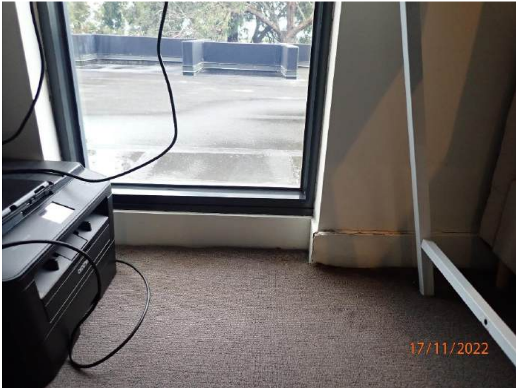
Photograph 51 - Apartment 417B bedroom 2 west facing window
