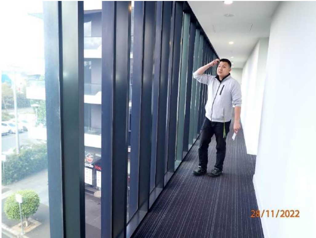
Photograph 81 – Level 4 south passageway aluminium windows
