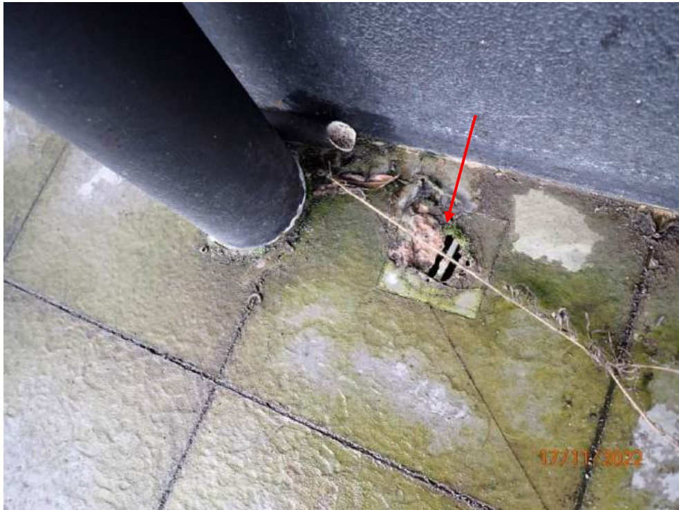
Photograph 19 - Apartment 308A balcony drainage outlet
