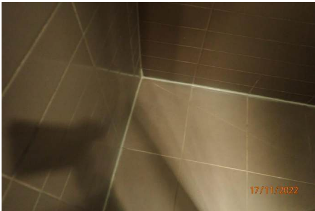
Photograph 122 – Apartment 521B bathroom shower, resealing of tiled floor perimeter
