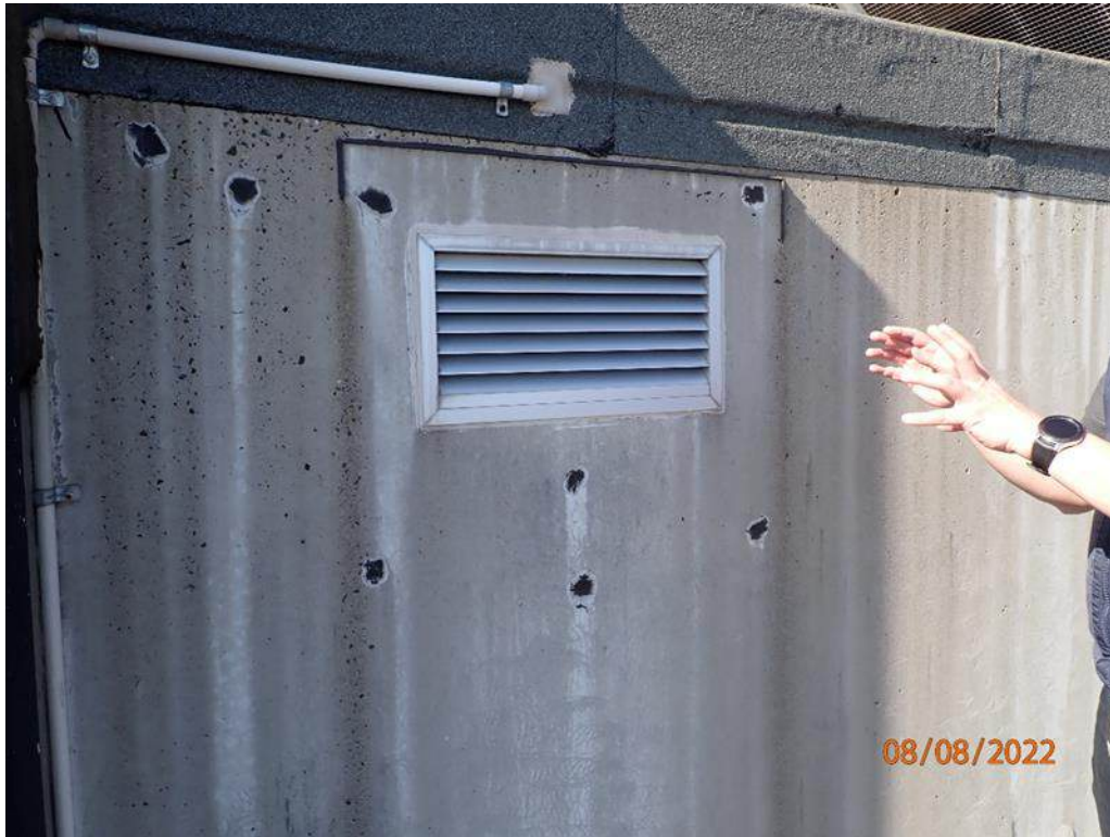
Photograph 137 – Building A, rooftop level, air vent to west wall of lift shaft
