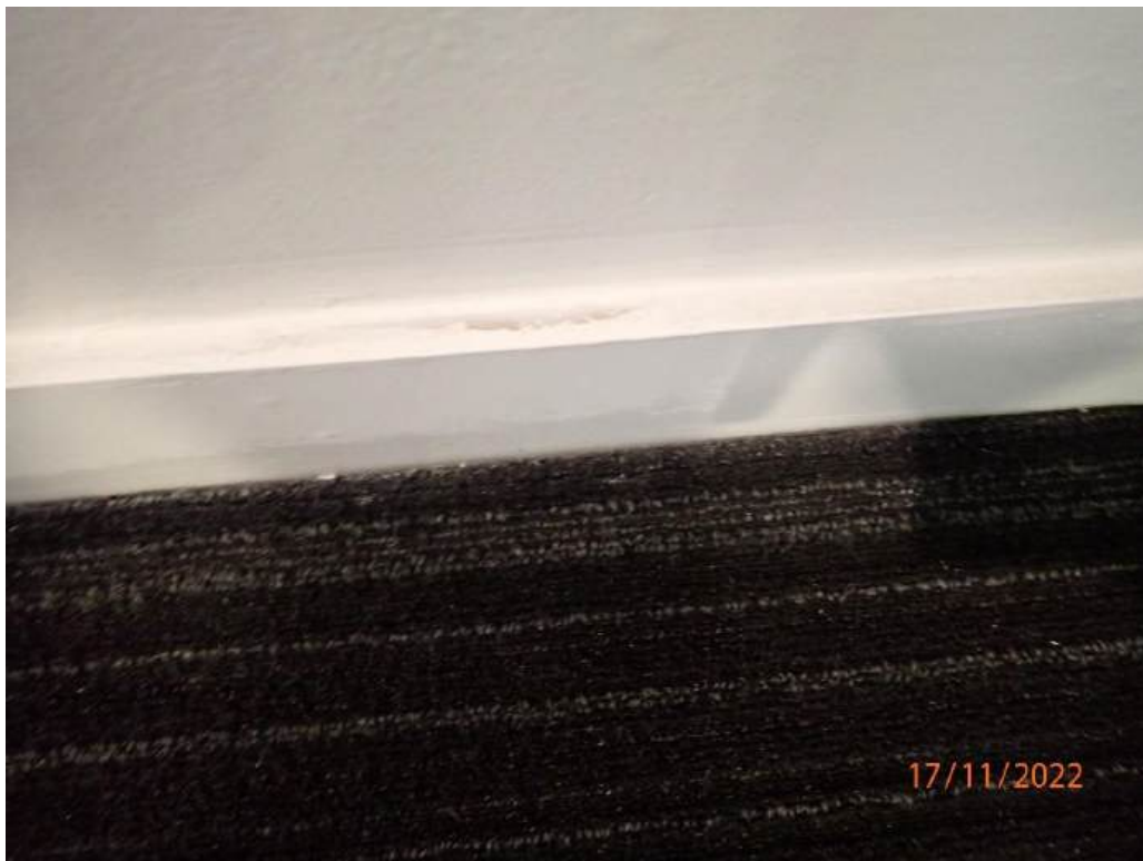
Photograph 42 - Common passageway outside Apartment 328B, recent repairs to plaster wall and skirting trim
