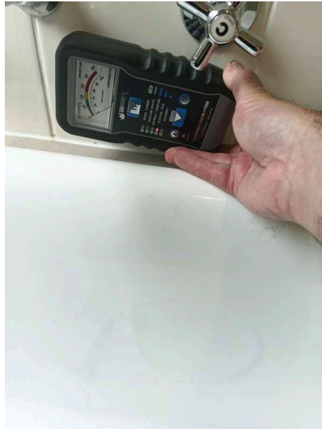
Toilet: Moisture reading to wall at toilet water supply tap
