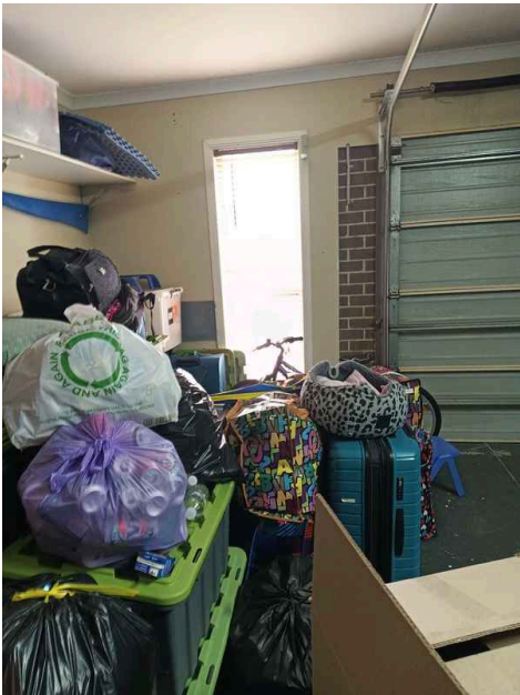
Window Conditions: General View
