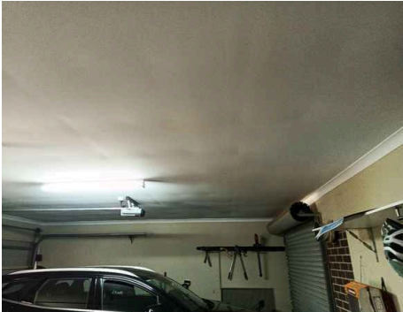
Ceiling Lining Condition: Ceiling General View General wear and tear noted
