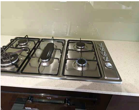
Range/Stove/Cooktop/Oven/Dishwasher: Oven General View
